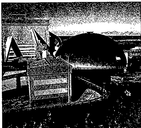
Kennecott Utah Copper's new smelter.
