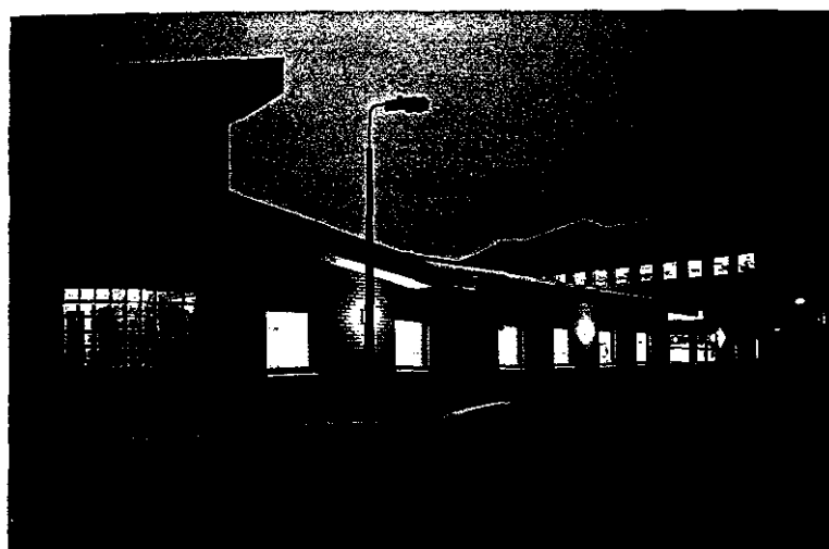
The new Brain Injury Rehabilitation Unit at Edgware Community Hospital.
