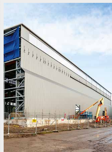
14,000m 2 of roof sheeting and wall cladding used to complete the press house
