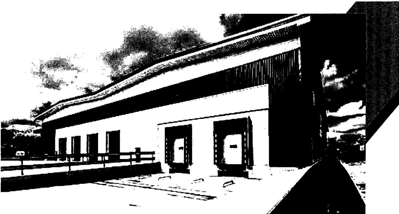
Pictured: MV55 is a 55,000 sq ft warehouse located at Markham Vale, a 200-acre industrial and logistics development located at Junction 29A of the M1 in Derbyshire.
