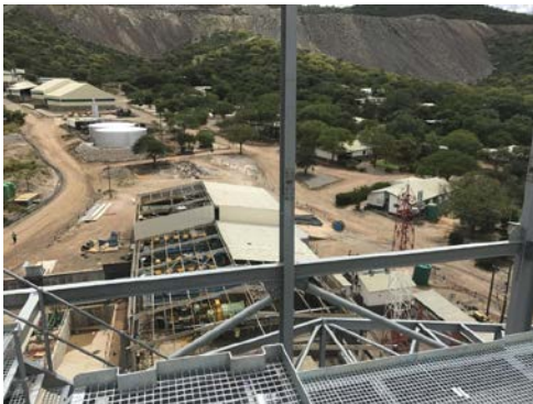
Gecko-Imerys Graphite Processing Facility
