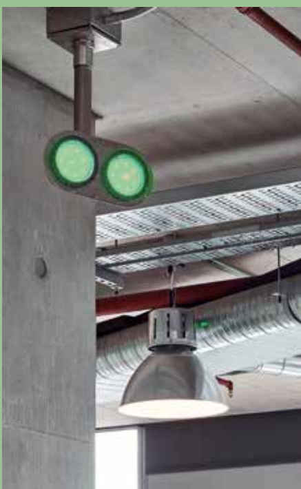
Above: White Collar Factory EC1: Traffic light building management system to denote windows are openable to allow for natural ventilation
