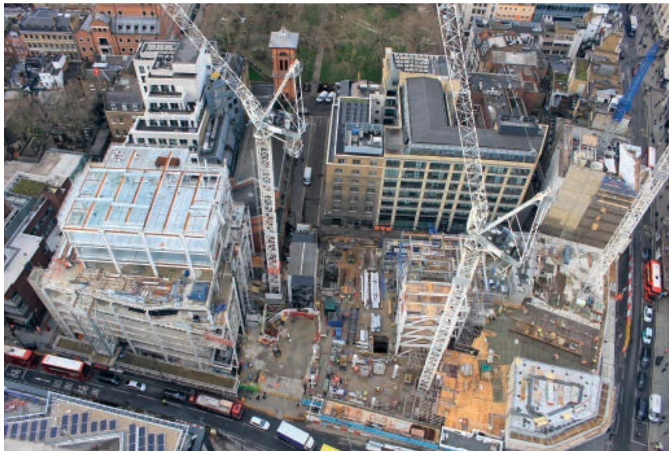
Soho Place site
