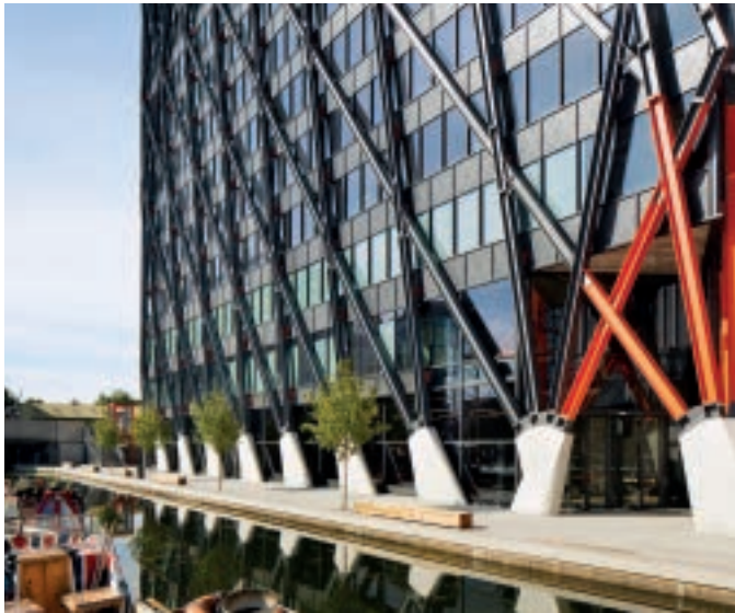
Brunel Building W2 – completed in May 2019
