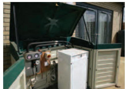
Ground source heat pump at Ravenswood, Ipswich, Suffolk and high thermal "U" valves meant homes complied with Code level 4
