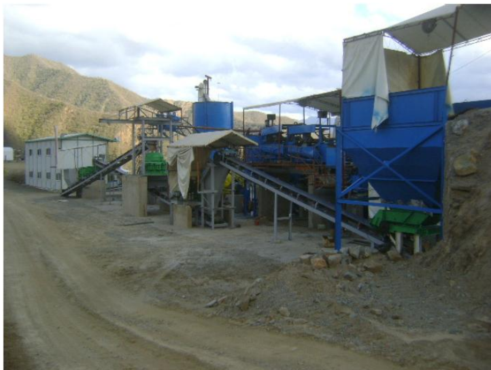
Figure 13.4 Wider view of 16.3, showing horizontal vibrating screener along part of the ore bin. The mine office and lab appear in background.)
