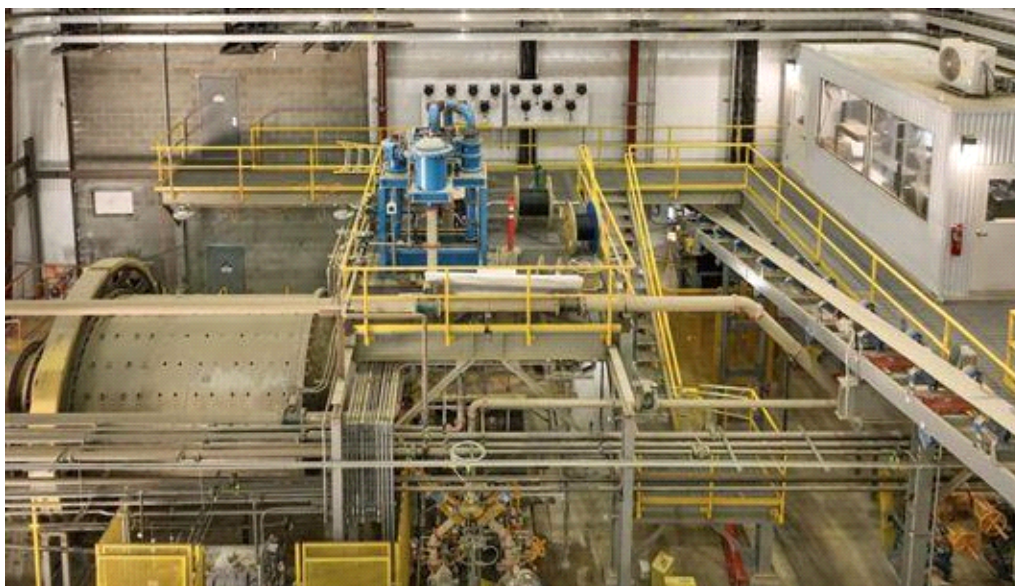
Figure 3: Process plant infrastructure at Bunker Hill advancing toward commissioning, supporting the planned June restart
