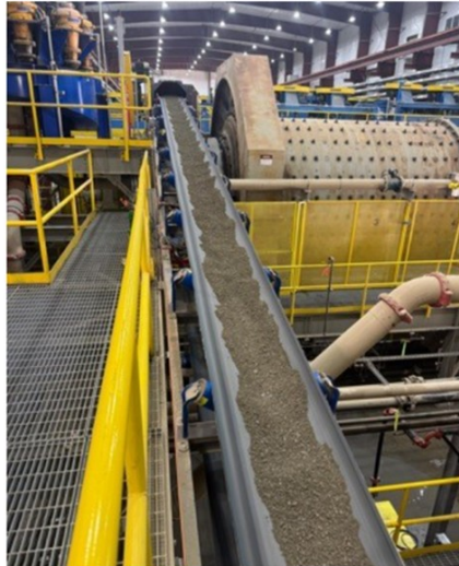
Crushed ore being taken by to main ball mill
