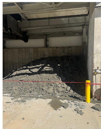
Filter cake ready to be transported to paste plant
