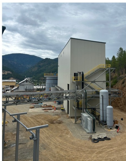
Tailings Filter Press Building
