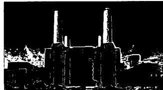
Battersea Power Station fire suppression systems
