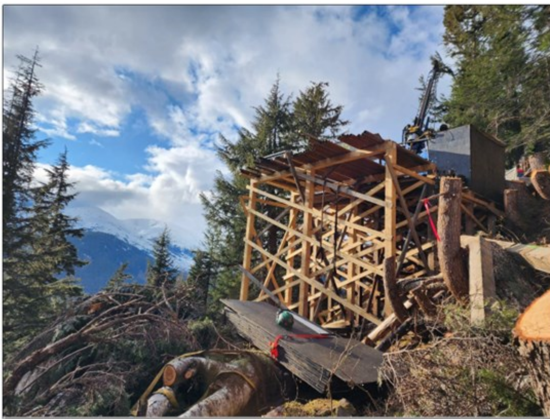
Figure 4. The 2025 Drilling Program started mid-May at Dolly Varden Silver's Kitsault Valley Project due to low snow accumulation; pictured is one of four drills currently drilling in the Kitsault Valley.
