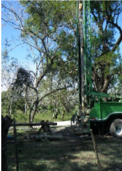
Photo 20.5 - Installation of a Water Well in El Ojital Community Source: ERM (2012)
