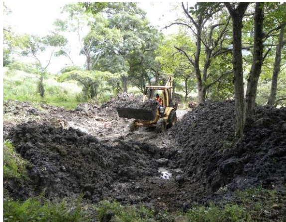
Photo 20.4 - Building of a Dam as Part of the "Infrastructure" Program Source: Provided by Minera Cardel (2012)
