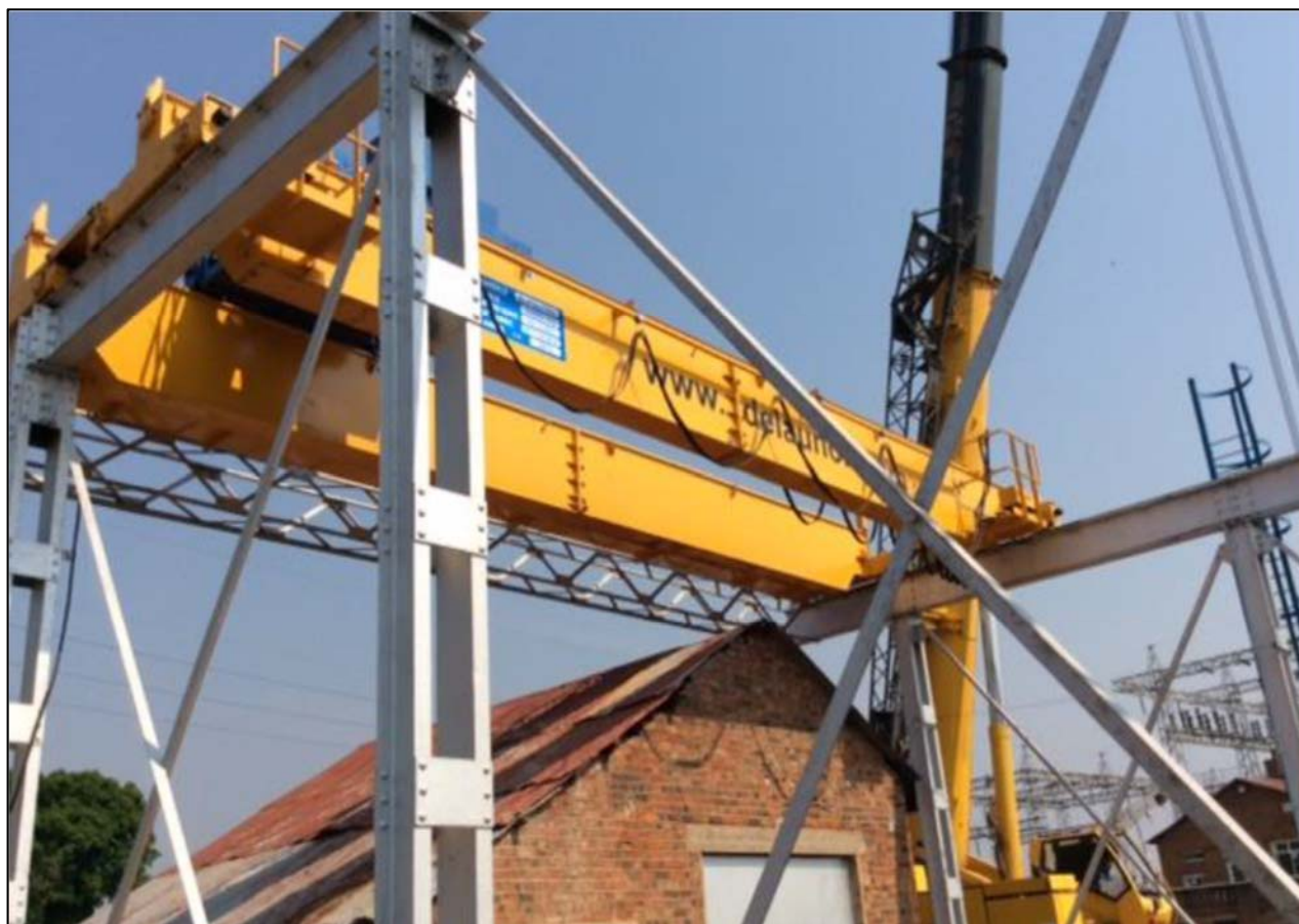
Figure 4: Mechanical installation of four overhead cranes completed at the Mwadingusha hydroelectric plant.
