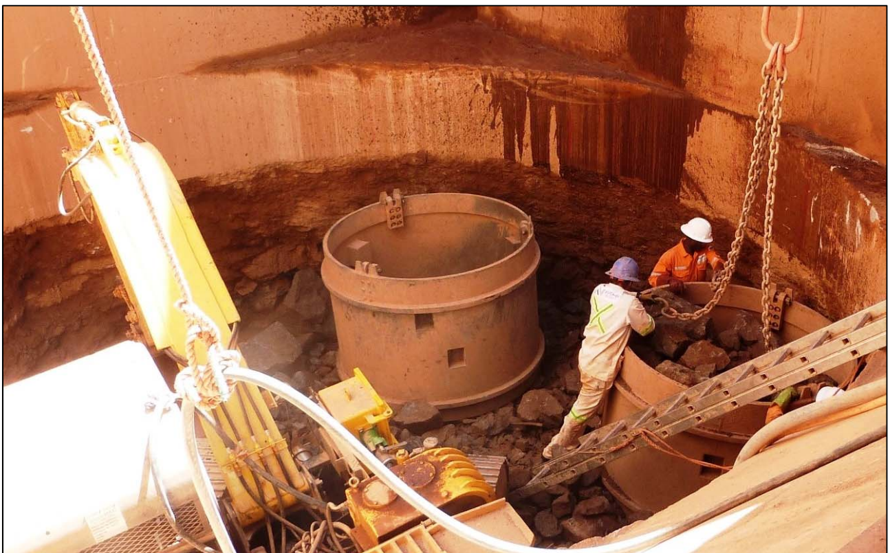
Figure 7: Initial sinking activities at Shaft 1 bottom.
