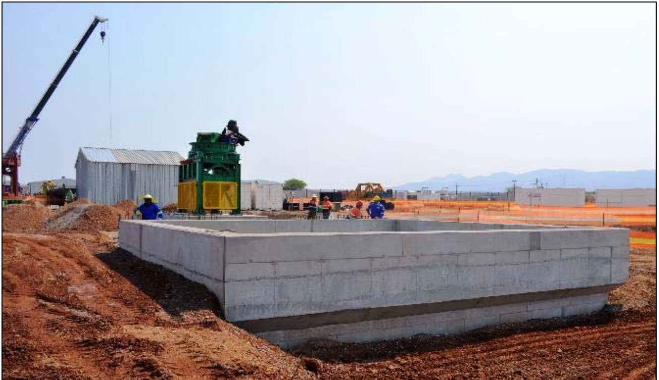
Figure 7: Initial sinking activities at Shaft 1 bottom.
