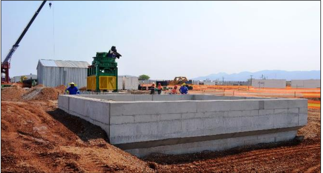
Figure 6: Top of Shaft 1 collar and pre-sink winder installation.
