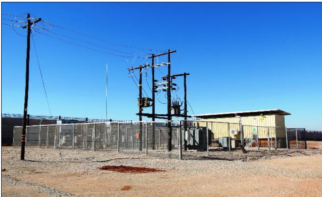
Figure 9: Construction of a 5MVA substation at Platreef is complete.
