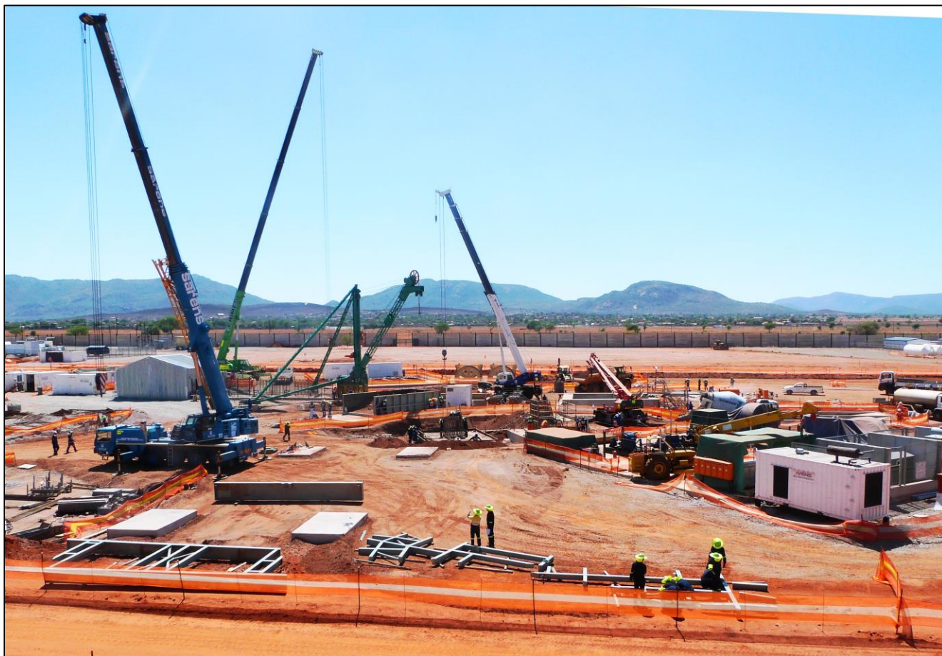
Figure 8: Overall view of Shaft 1 works.
