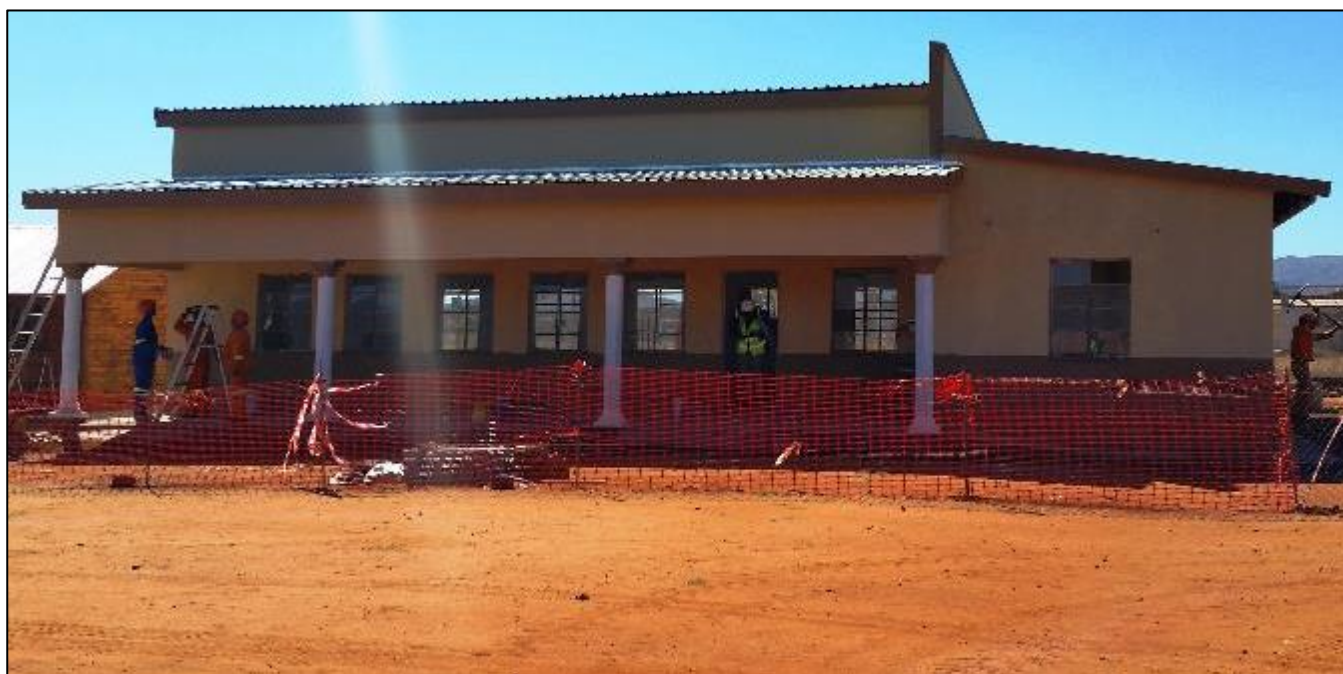
Figure 10: Renovation of a local community care centre.
