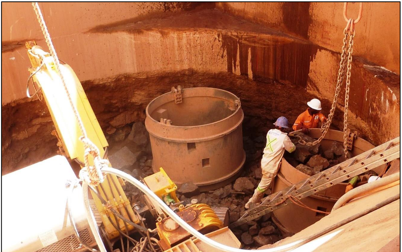
Figure 7: Initial sinking activities at Shaft 1 bottom.
