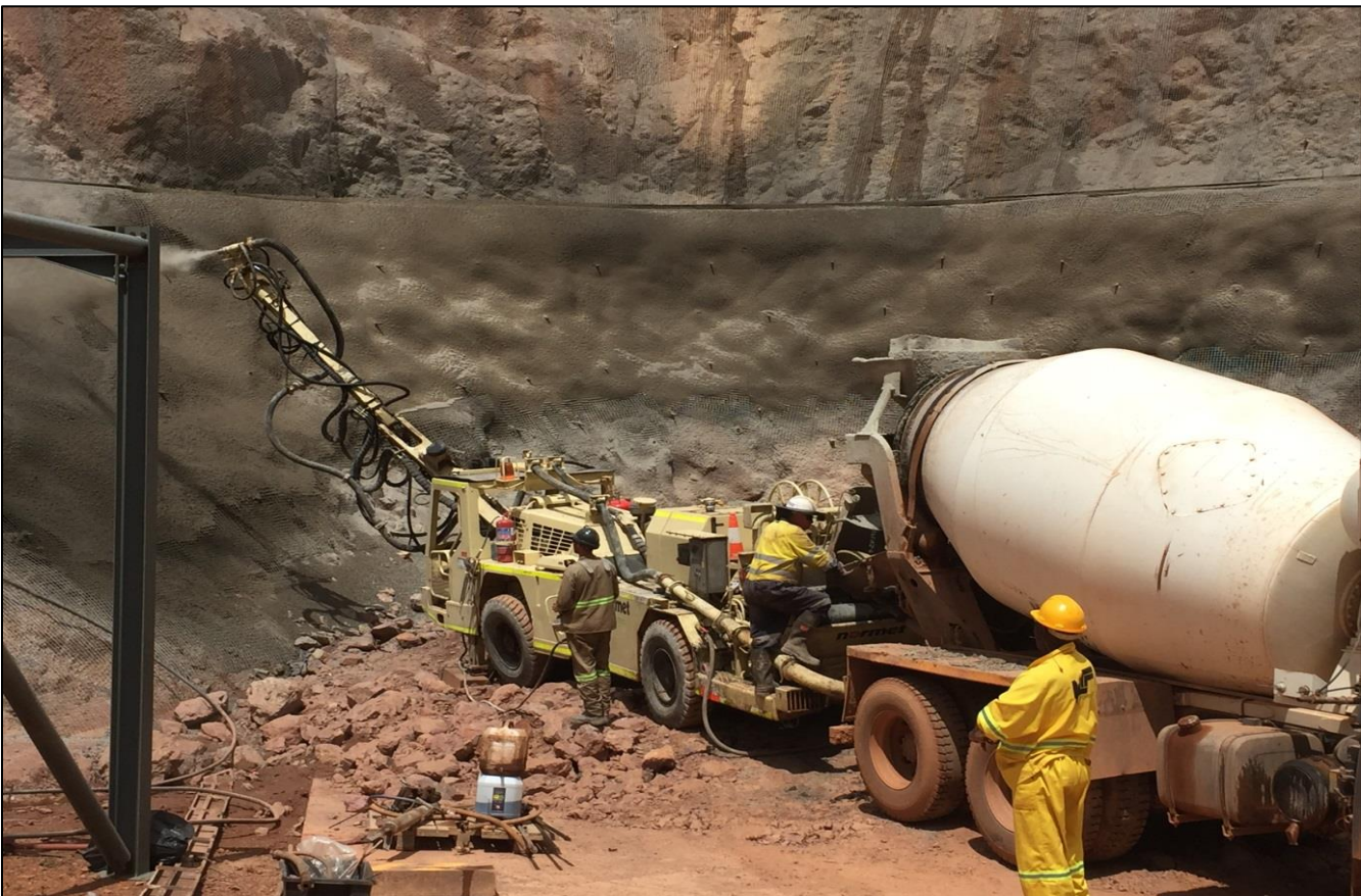
Shotcrete application on the bottom bench.
