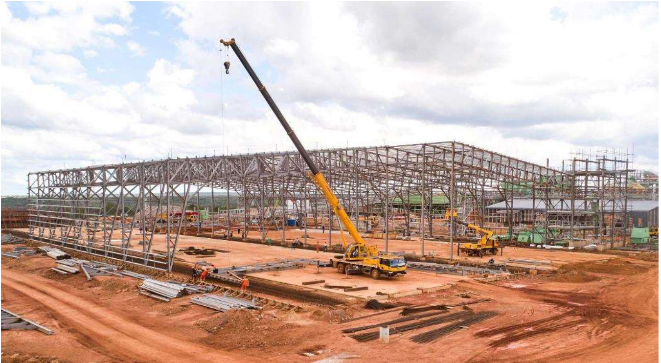
Workers installing a section for the two, 2,000-tonne silos at the backfill plant.
