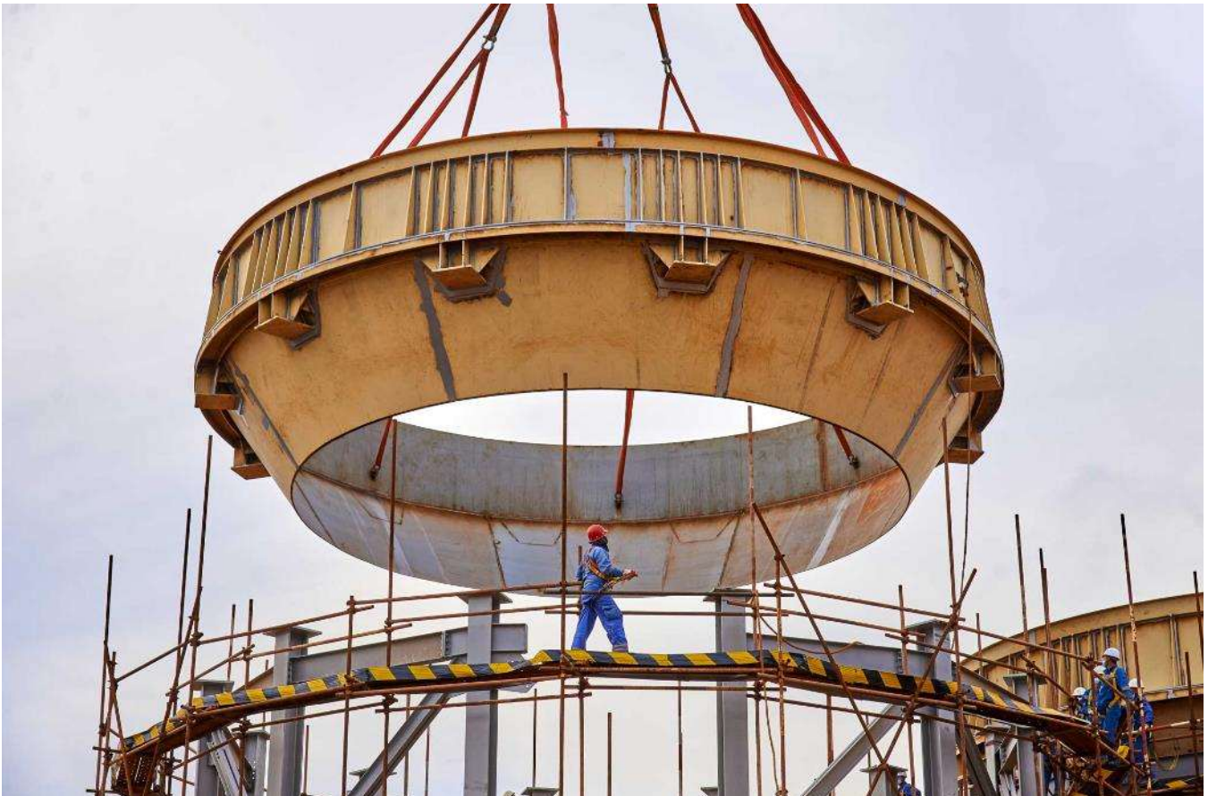
Workers installing a section for the two, 2,000-tonne silos at the backfill plant.
