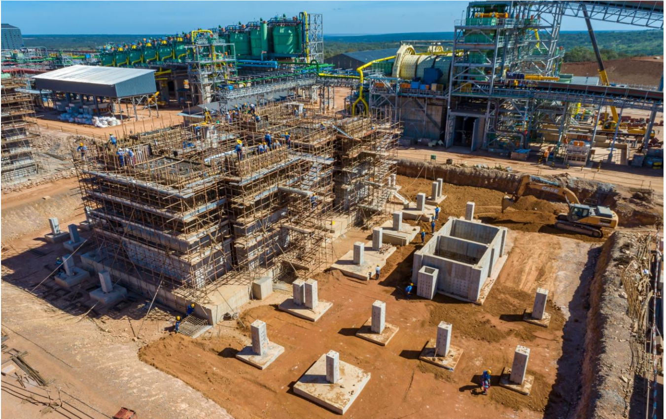
Construction of foundations for the Phase 2 high pressure grinding rolls.
