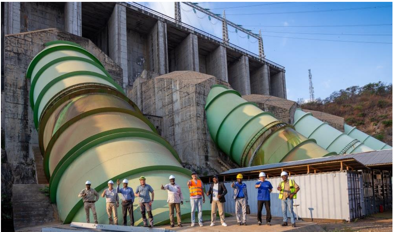
Engineers from Kamoja Copper, SNEL, Stucky and Voith Hydro at the 8-metre diameter penstock for turbine 5.
