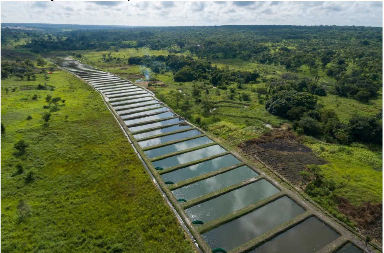
Photo: Newly constructed fish ponds near Kamoa-Kakula.
