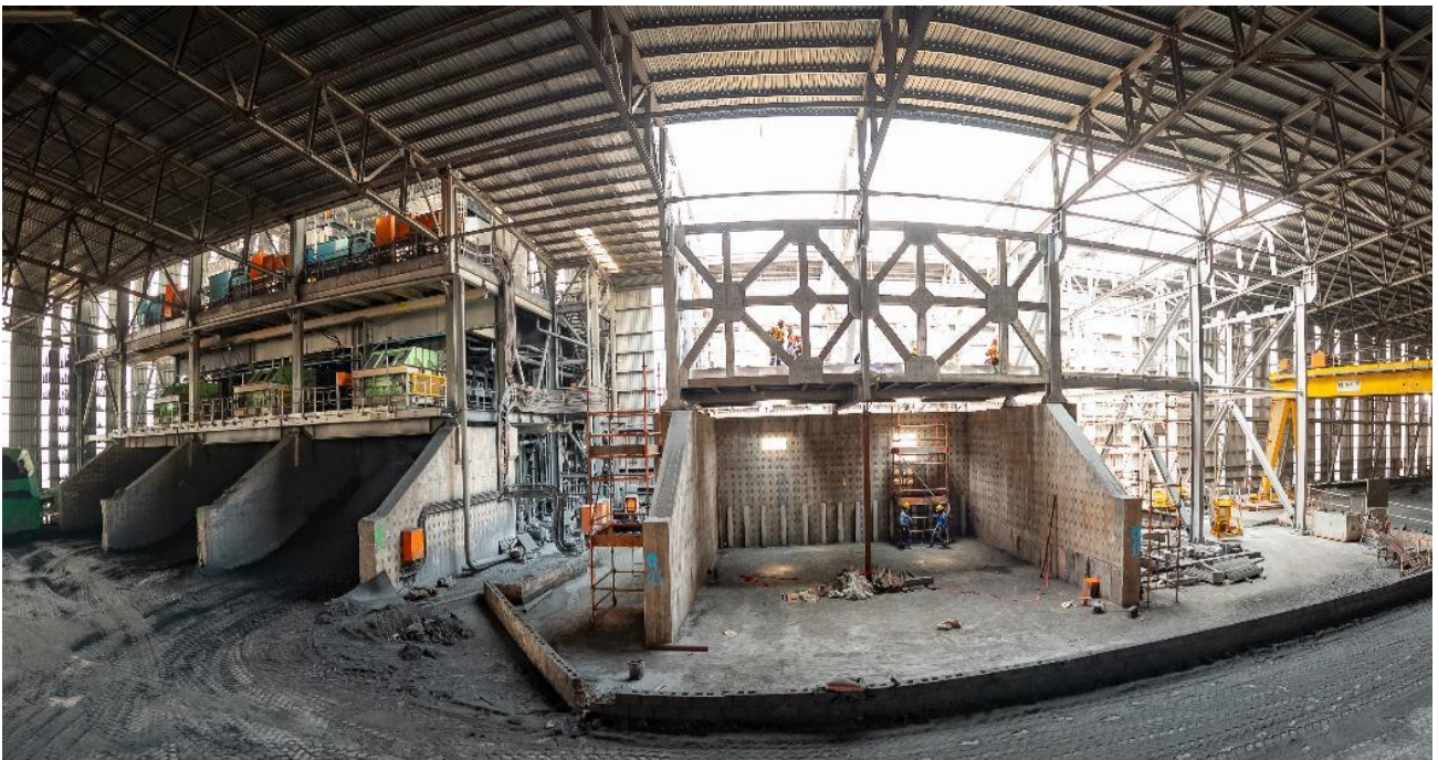
Photo: Construction is progressing well in advance of the installation of the fourth Larox filter press at Kamoakakula's concentrate warehouse.
