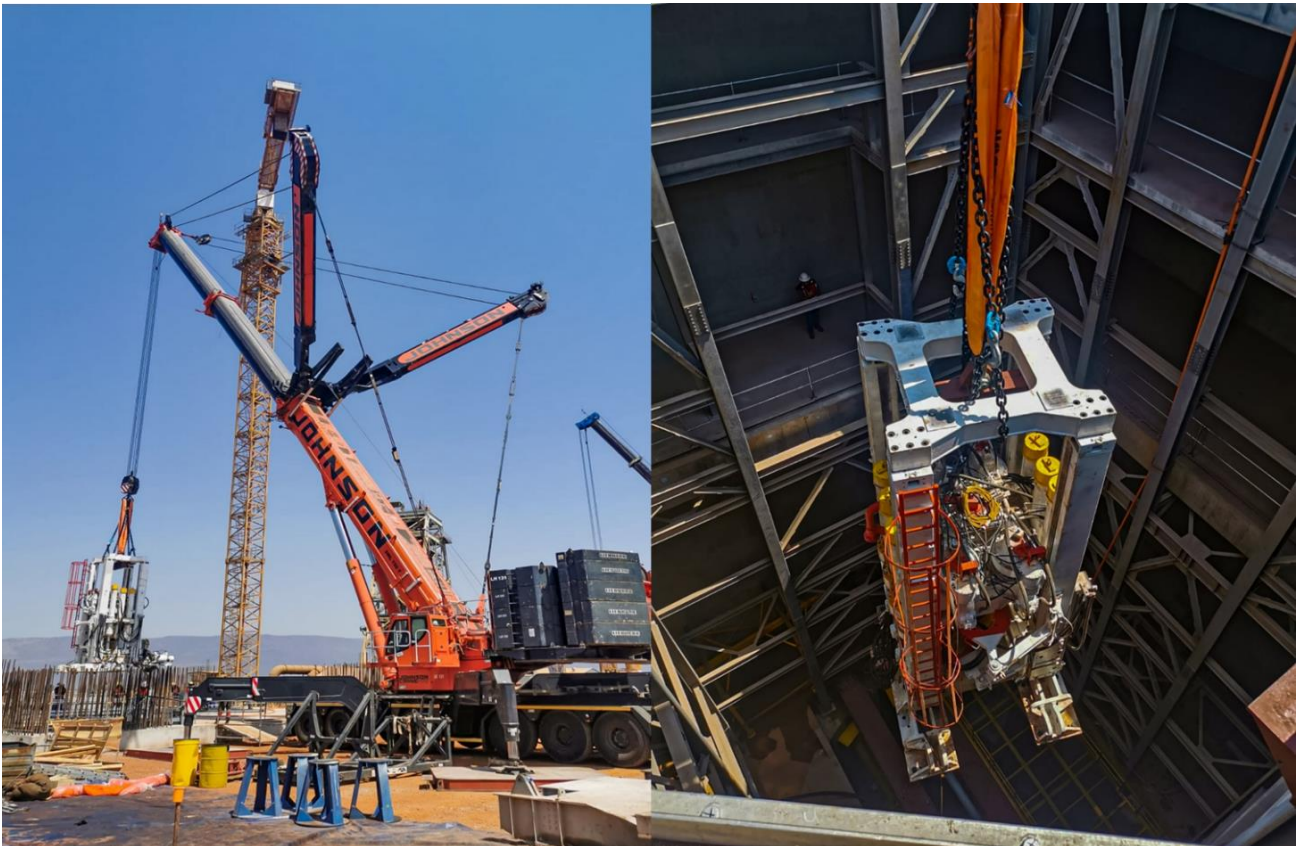
Photo: Shaft 2 raise-boring equipment being lowered into position.
