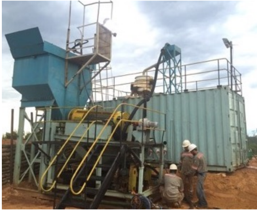
Bulk Sampling plant construction nearing completion at Jaibaras
