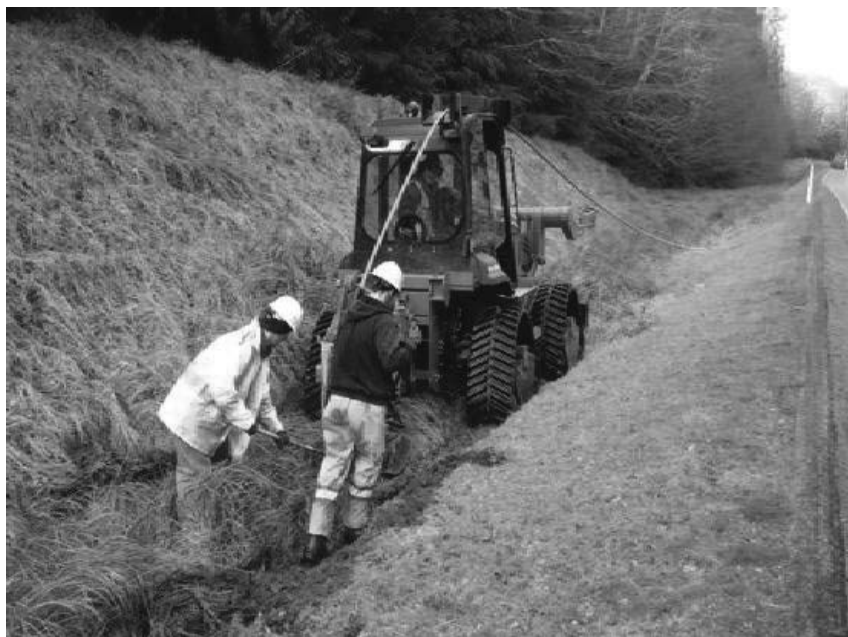
Figure 5: Vibratory plowing
