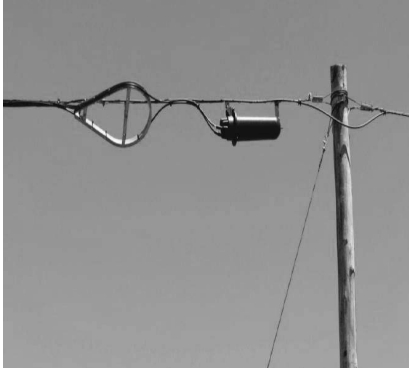
Figure 2: Ariel placement and splicing
