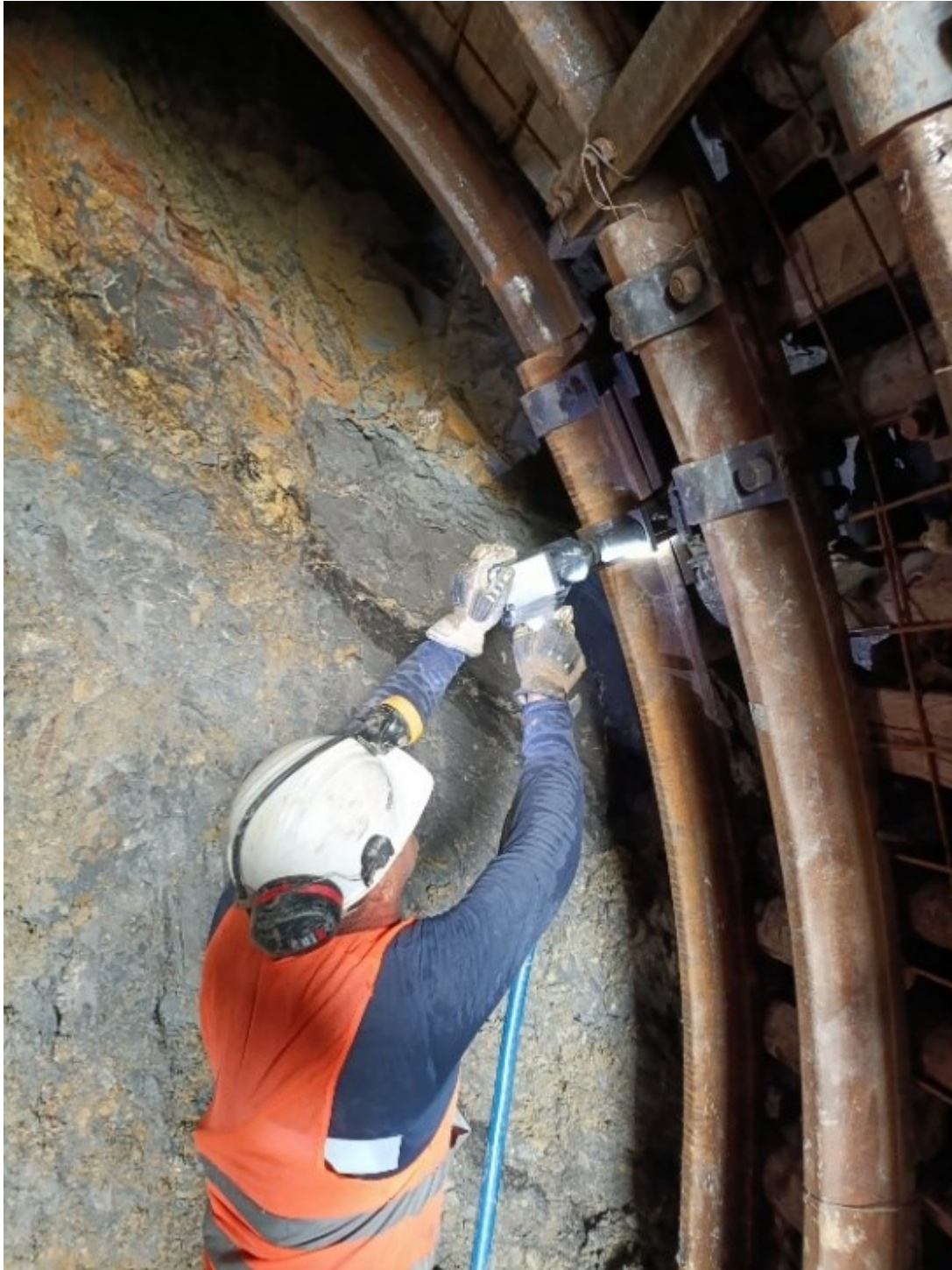
Figure 2. Worker torques fasteners on steel arches
