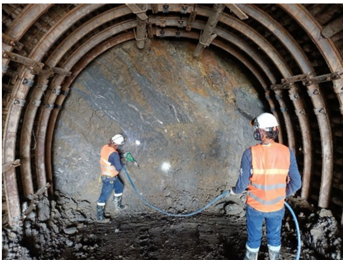
Figure 1. Workers scale rock from development face
