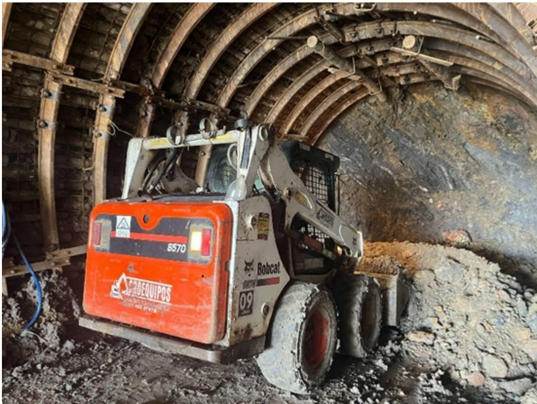
Figure 3. Muck being transported to the dump staging area
