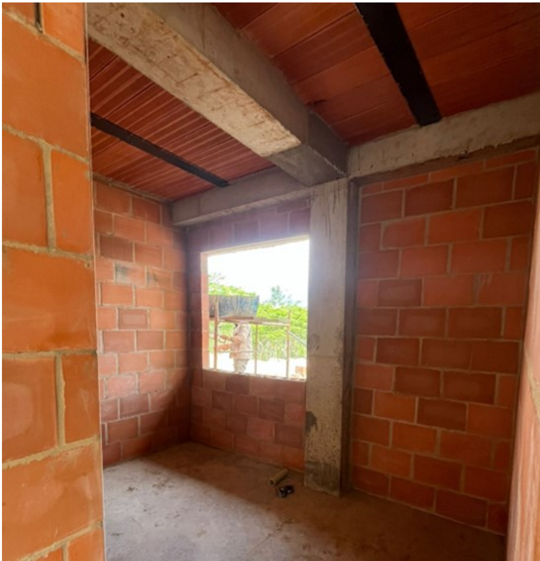
Figure 3. Interior of double occupancy camp accommodations
