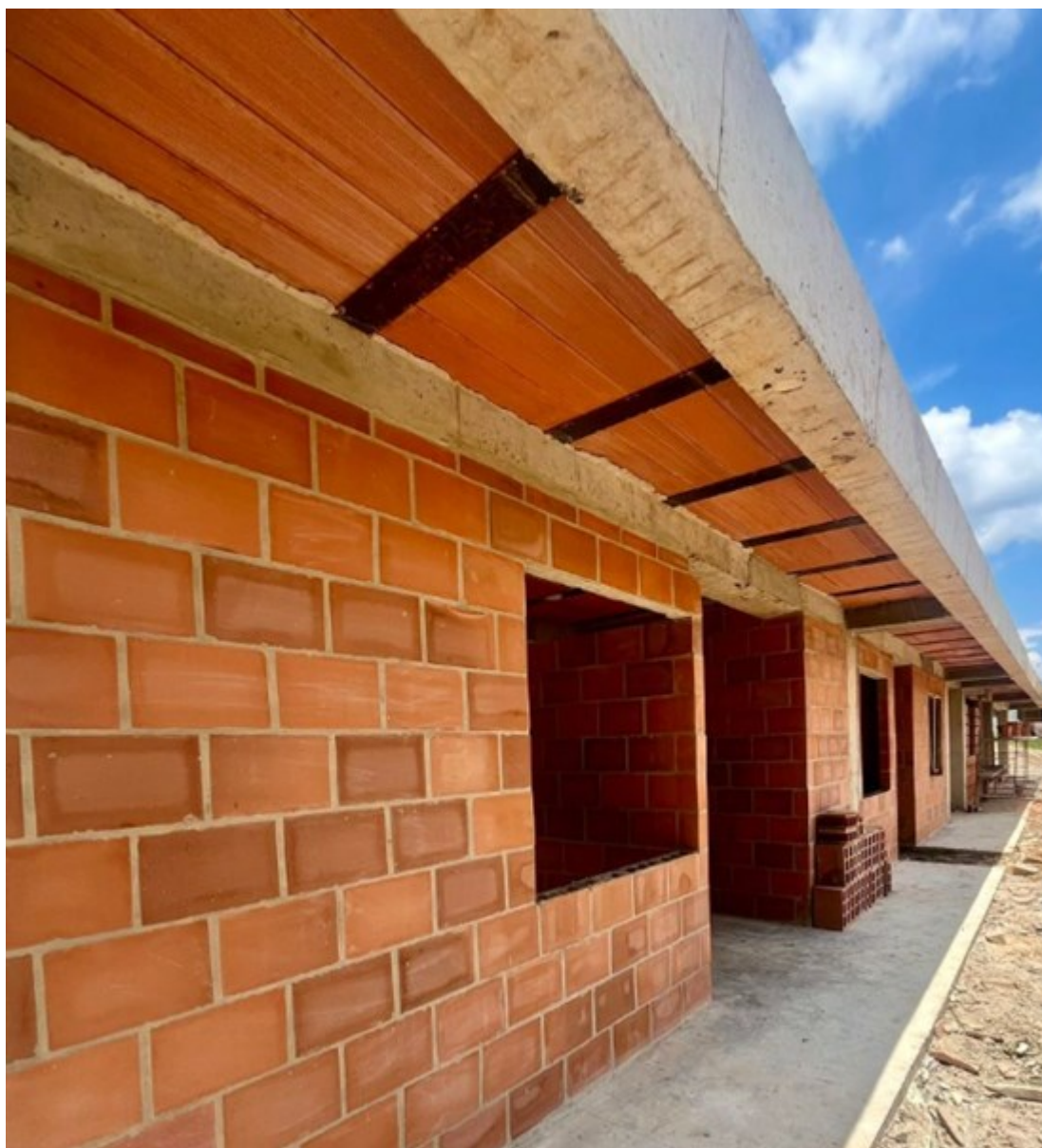
Figure 2. Exterior of camp under construction
