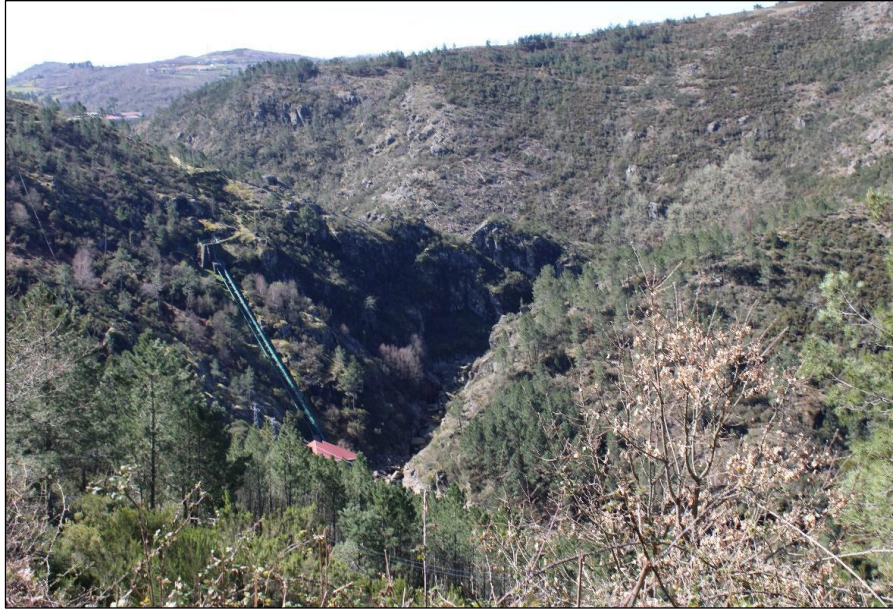
Figure 5-1: View looking northward at the Borralha Penstocks and Power Plant
