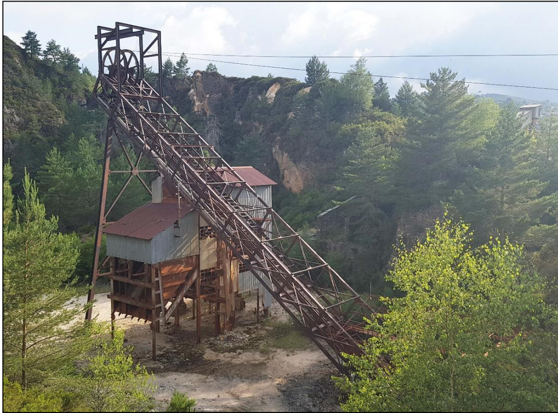
Figure 4-4: Inclined Production Shaft in the St. Helena Breccia Open Pit.
