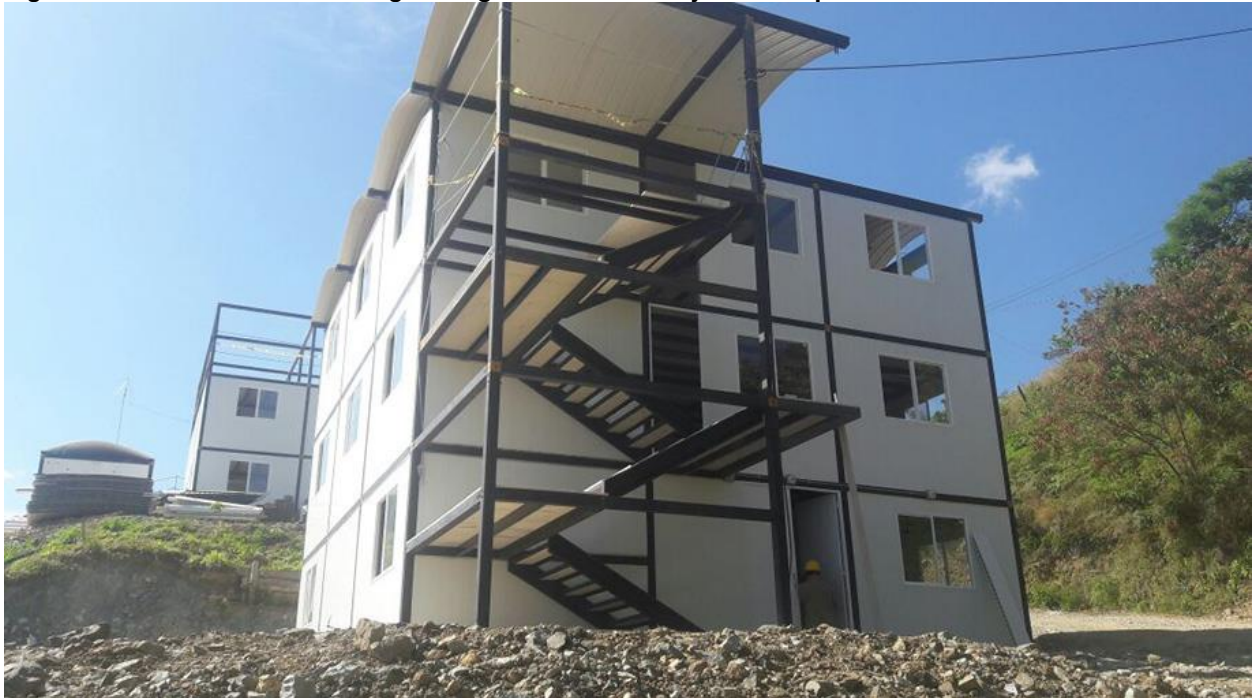
Figure 4: Modular Office Buildings being installed for Project and Operations Personnel
