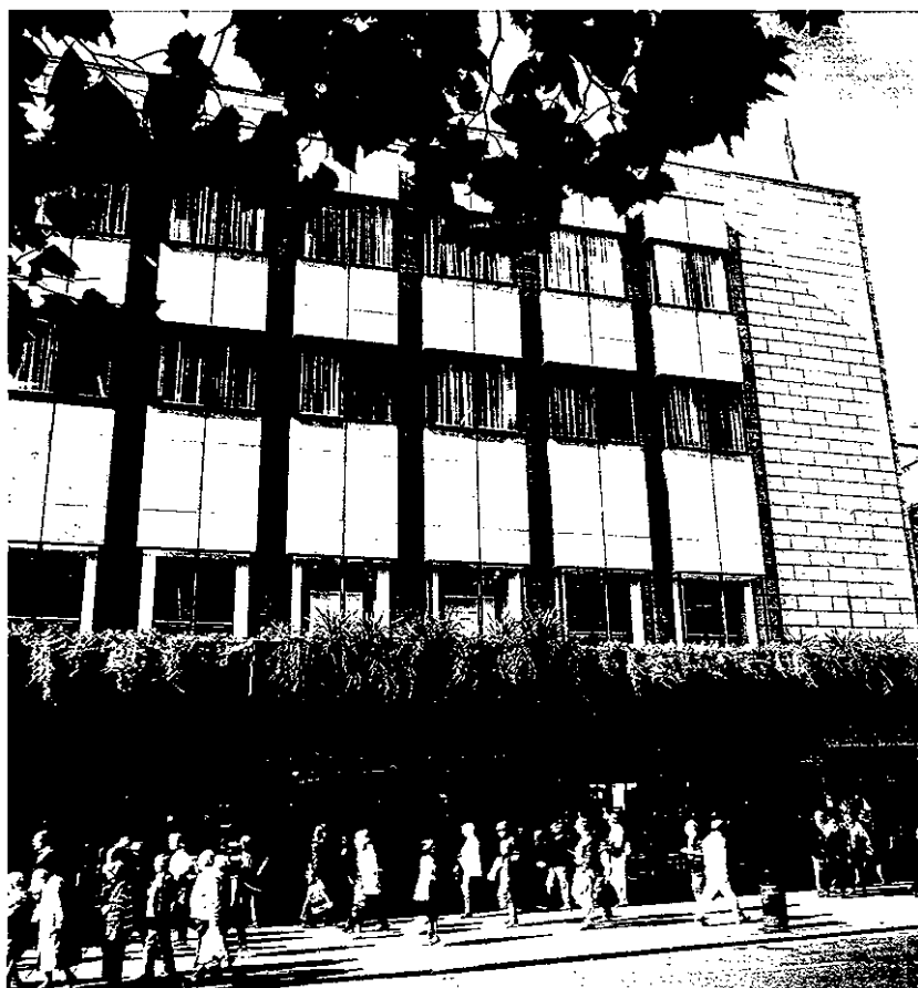
Penneys newly refurbished store at O'Connell Street, Dublin.
