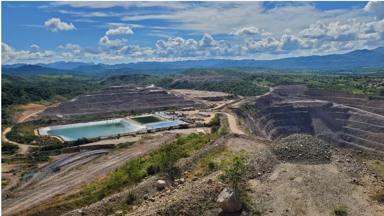
Figure 1: General View of the La Trinidad Mine and Surroundings
