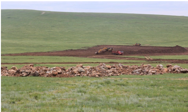
Pre-Stripping of ATO1 Deposit
