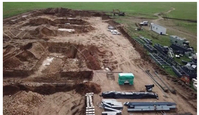
Crusher Construction Site
