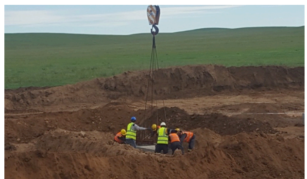
Crusher Footings Being Installed
