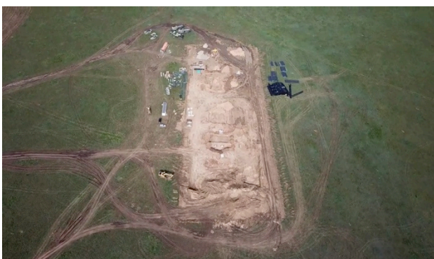
Crusher Construction Site
