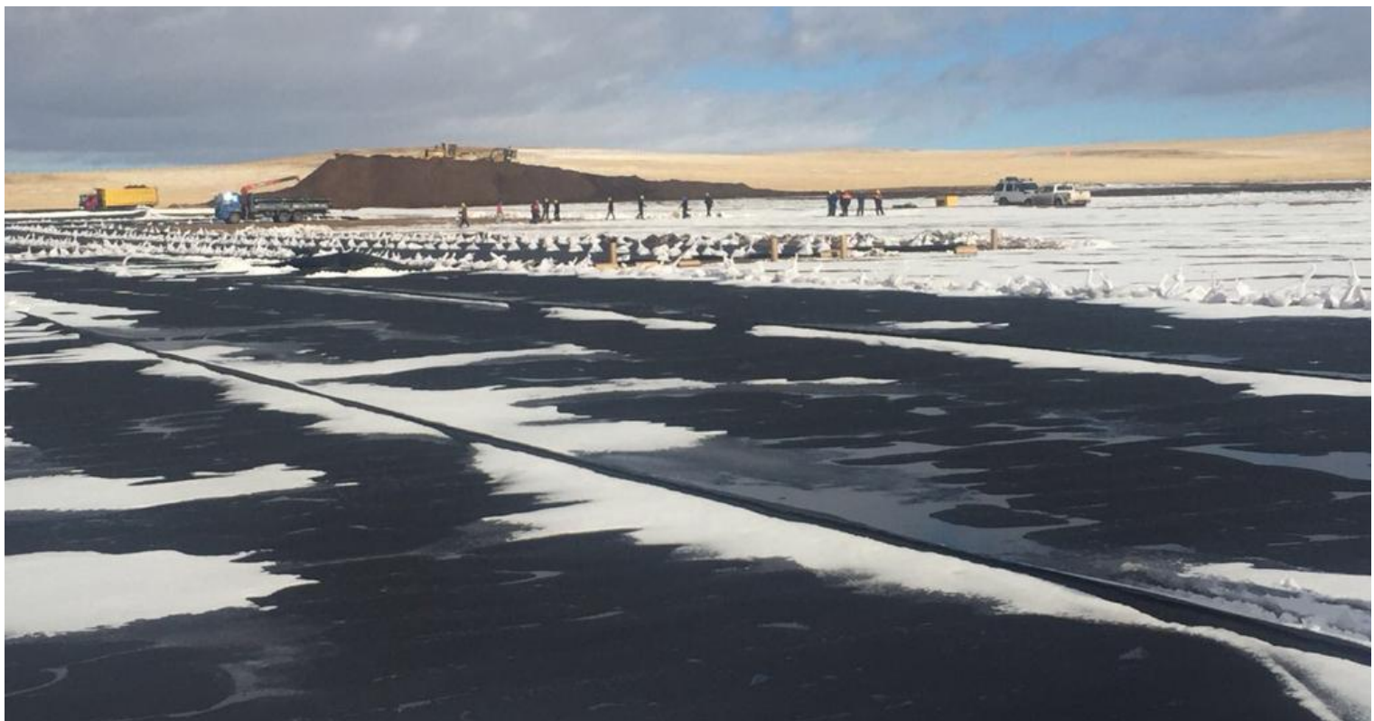
Liner being laid on cell 1
