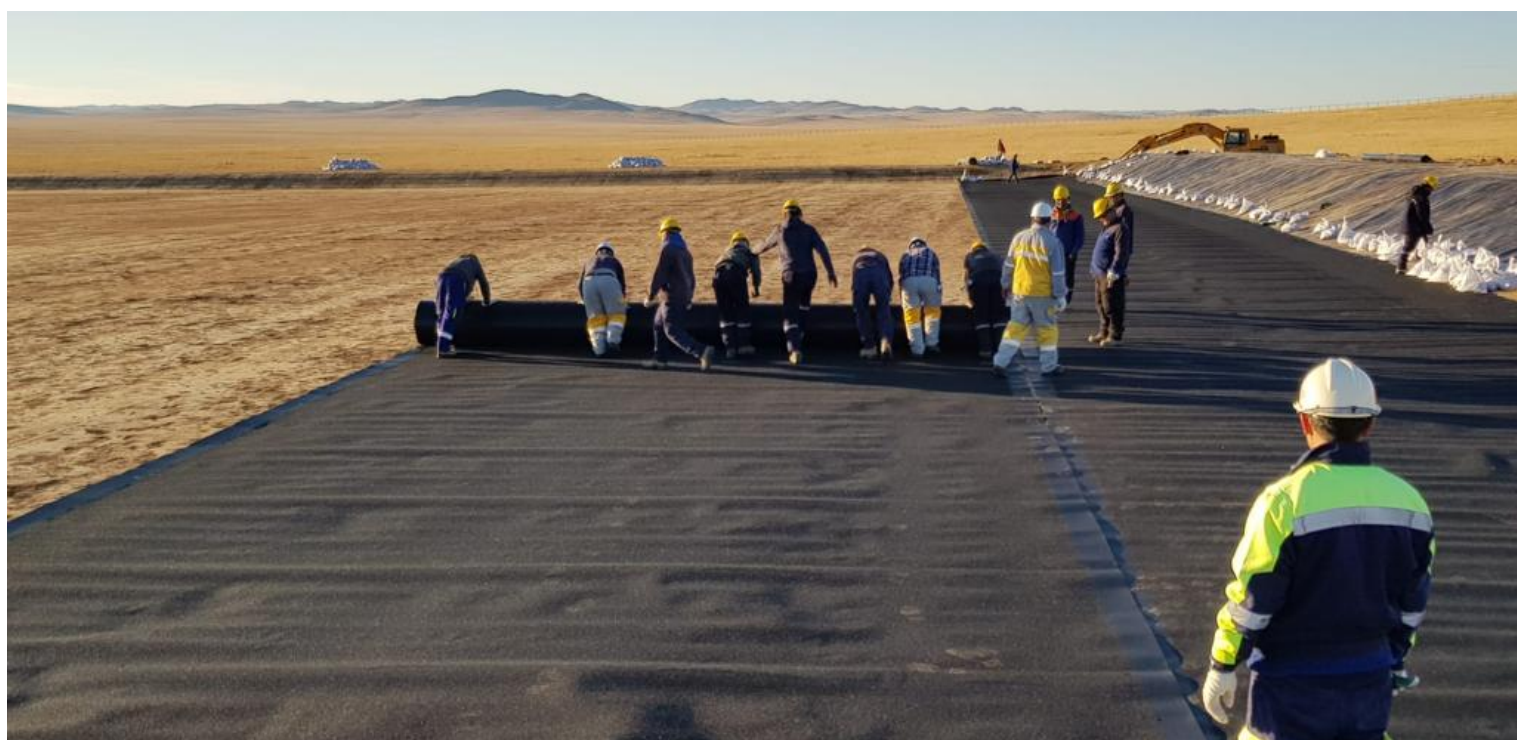
Cell 1 HDPE lining
