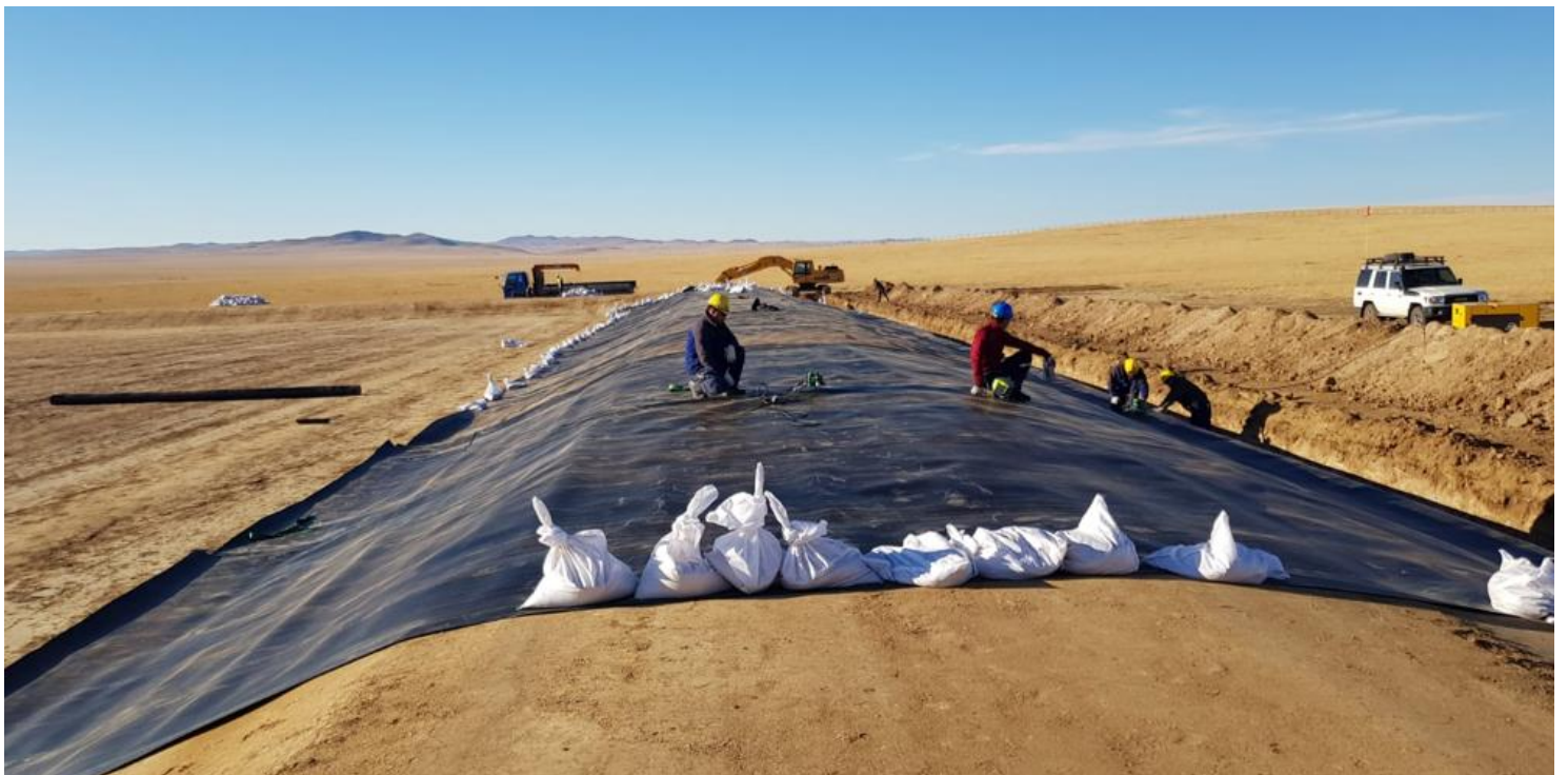
Cell 1 Embankment lining
