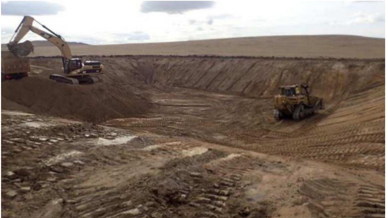
Barren & Pregnant Pond excavation
