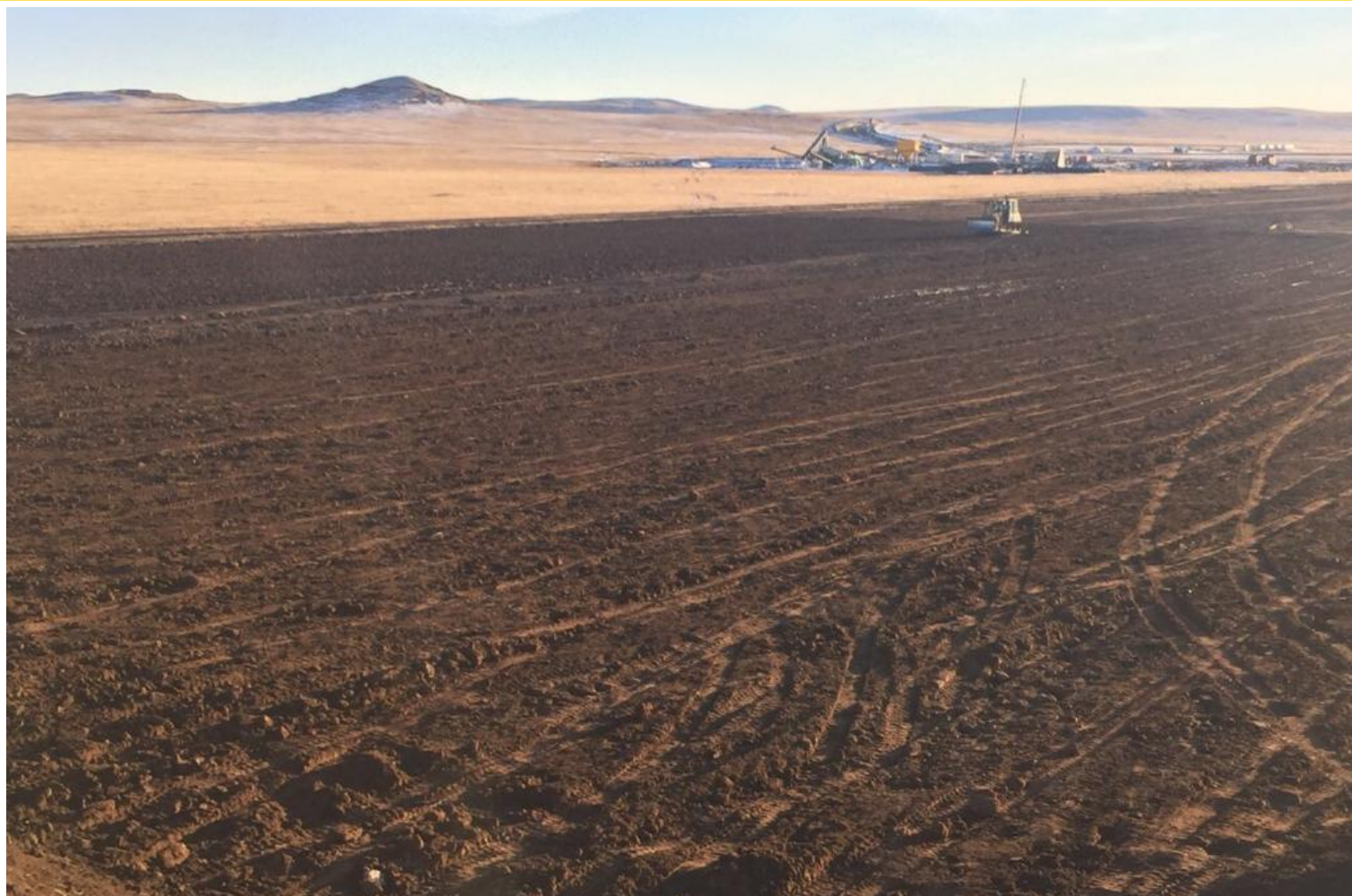
Cell 2 conditioning underway
