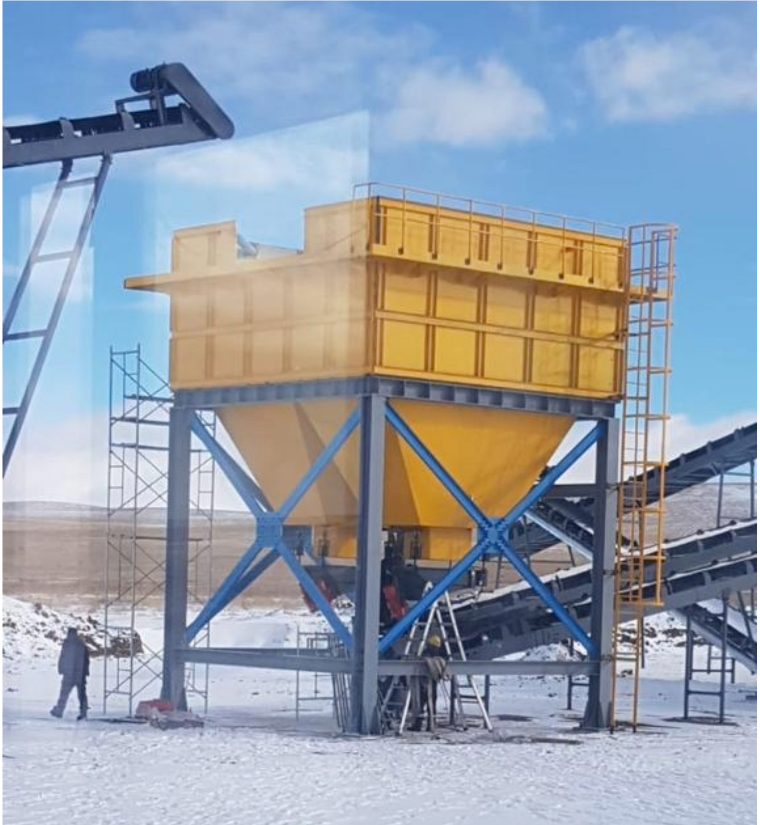
Hopper, bin construction complete
