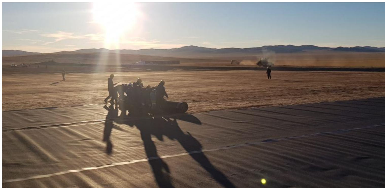
Cell 1 HDPE Lining continuing
