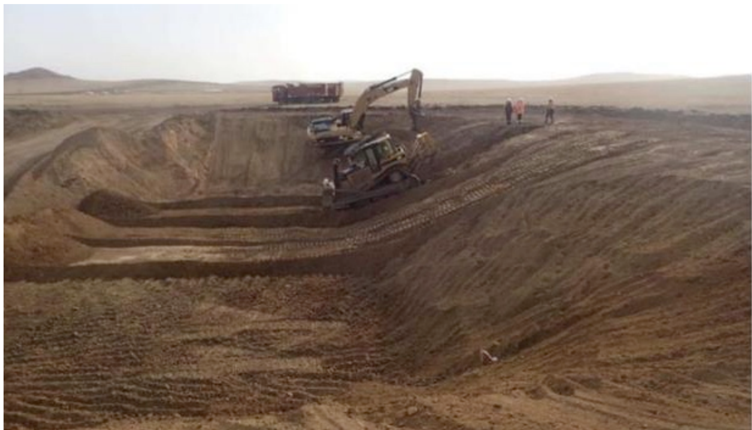
Barren & Pregnant Pond excavation
