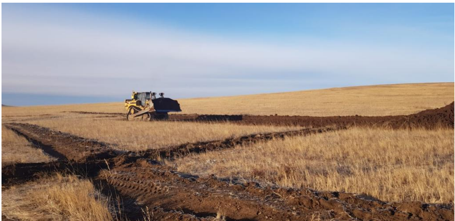
ADR Plant topsoil removal
