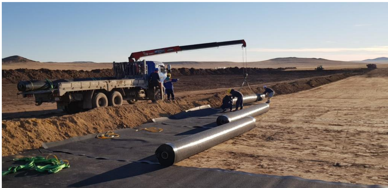
Cell 1 HDPE lining
