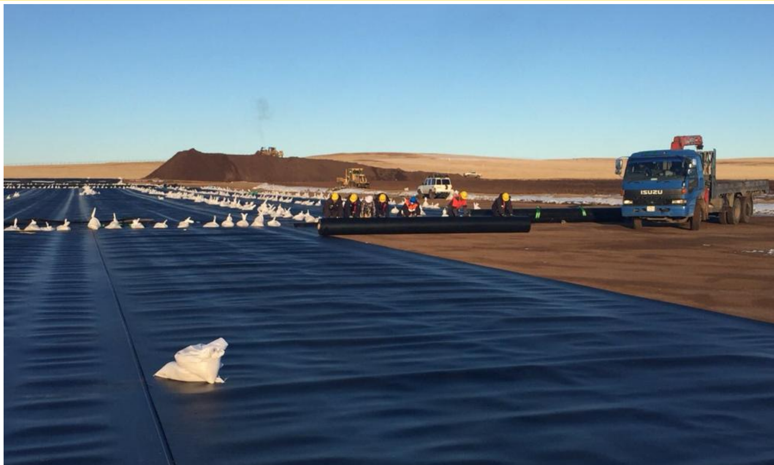
Liner being laid on cell 1
