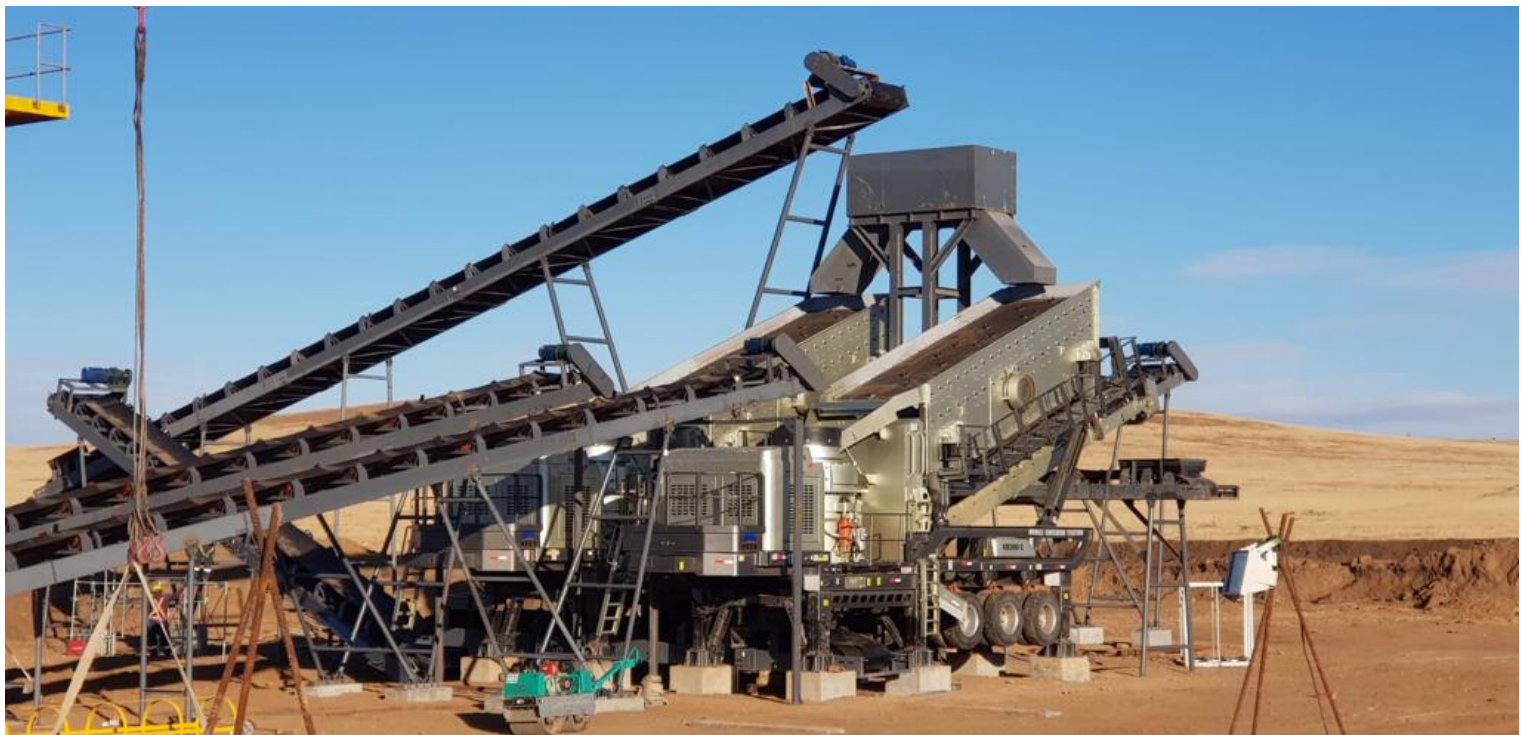
Cone Crusher construction
