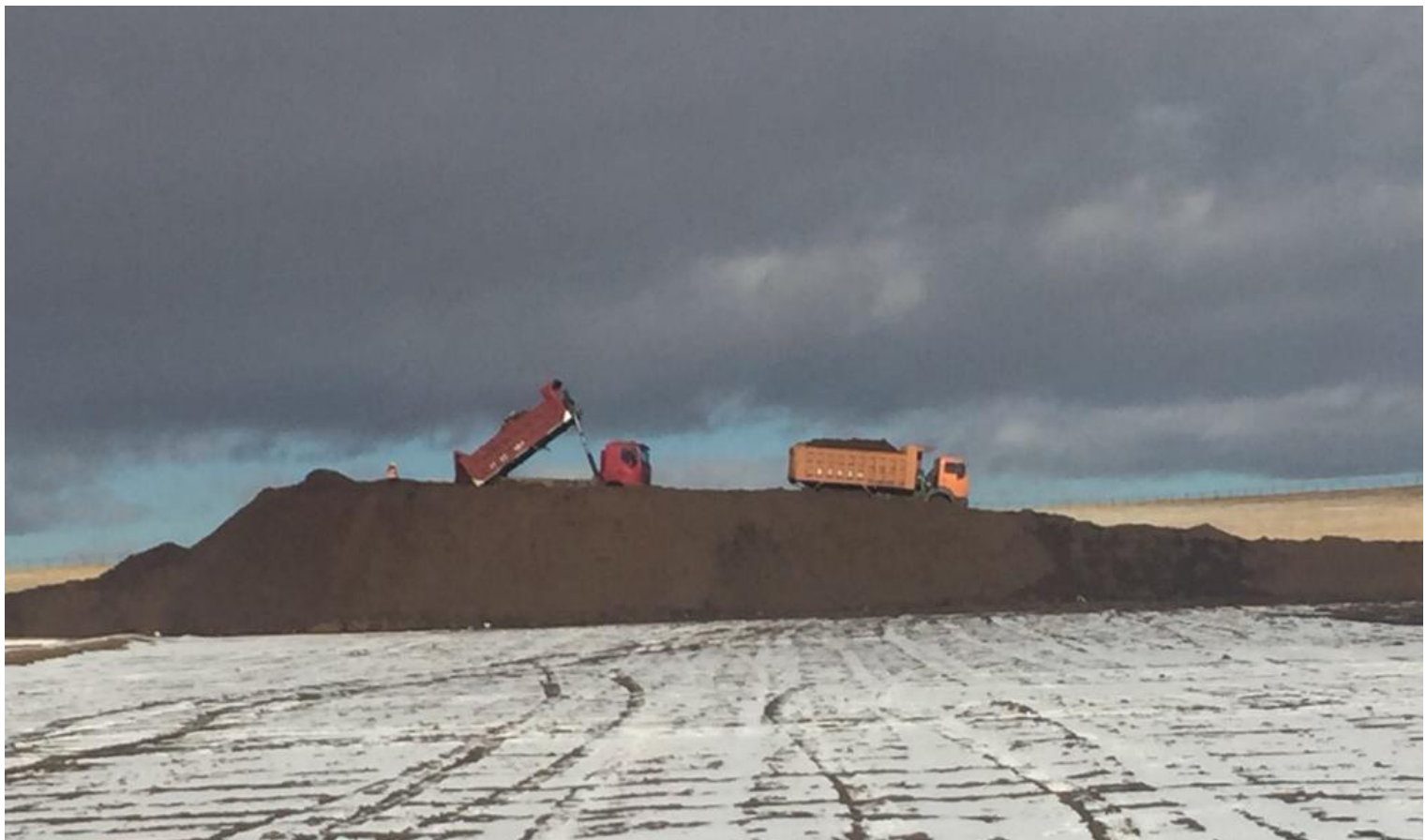
8 meter stacking ramp for cell 1 under construction
