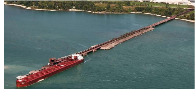
LEW Dock Infrastructure (Current)
