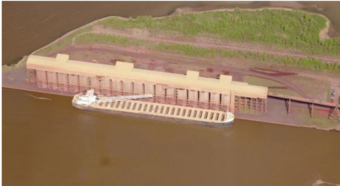
Figure 18-3: Allouez Taconite Facility Ship Loader and Silos
