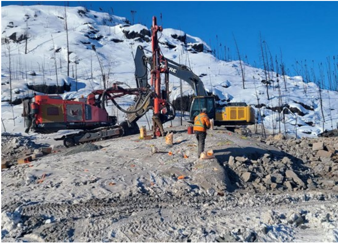
Preparing the blast for the mill foundation
