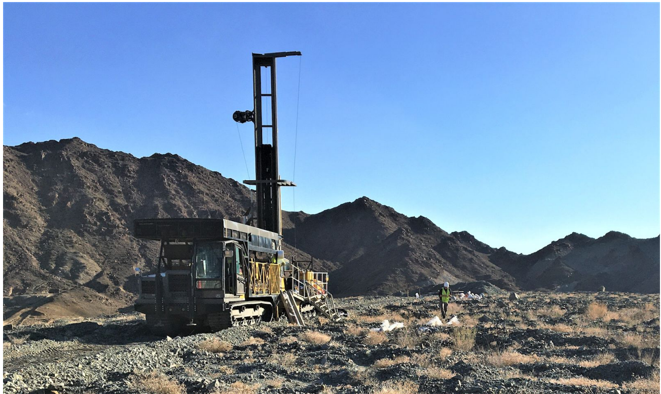
Sonic drill rig of Yellow Jacket Drilling Services, LLC on the American Girl historical heap leach pad (hole AGS-01)
