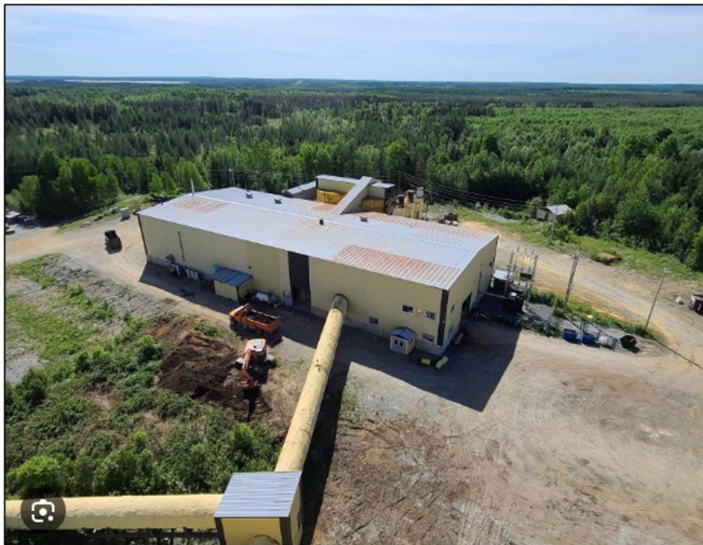
Figure 3: Photo of exterior of Beacon Mill in Val-d'Or, Québec
