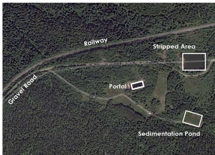
Figure 74 - Aerial Photo of Rehabilitated Swanson Site (Google Earth 2025)
