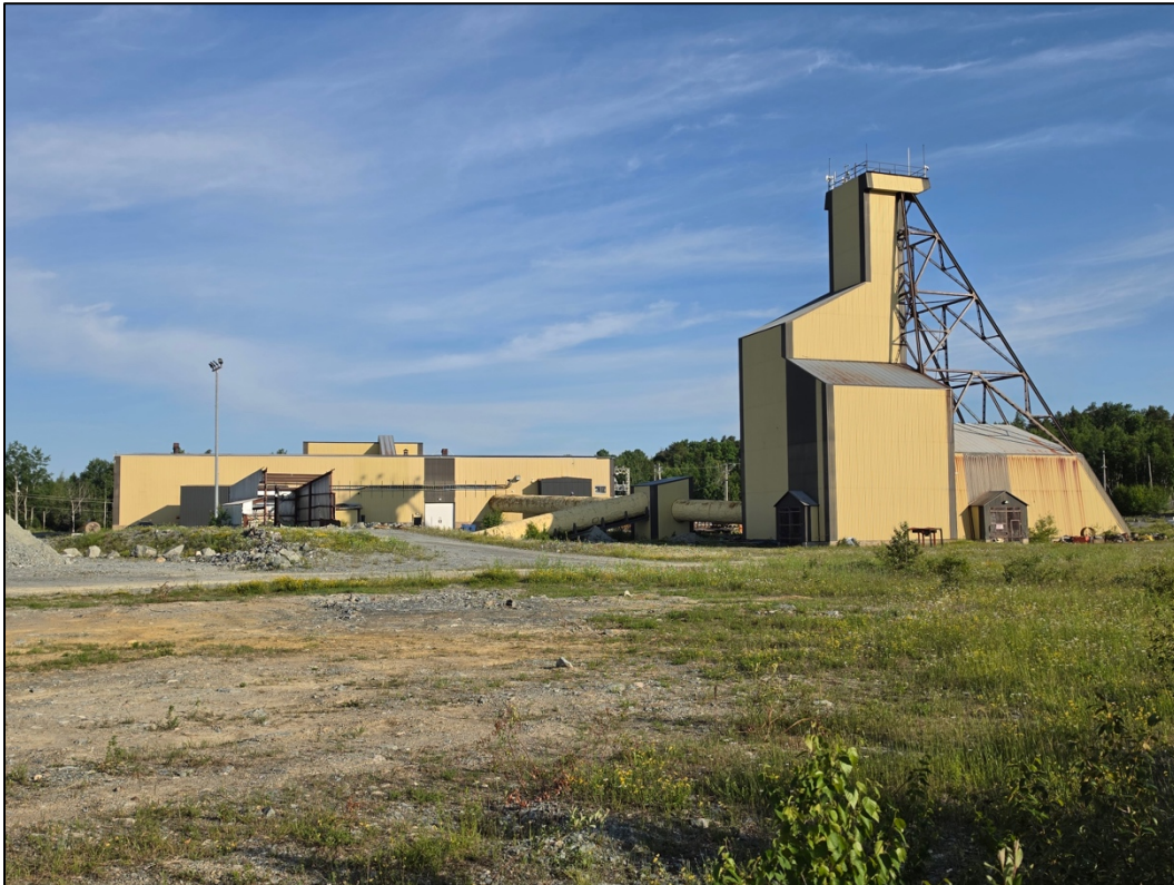
Photo 3: Exterior of Beacon Mill facility including covered conveyor and headframe
