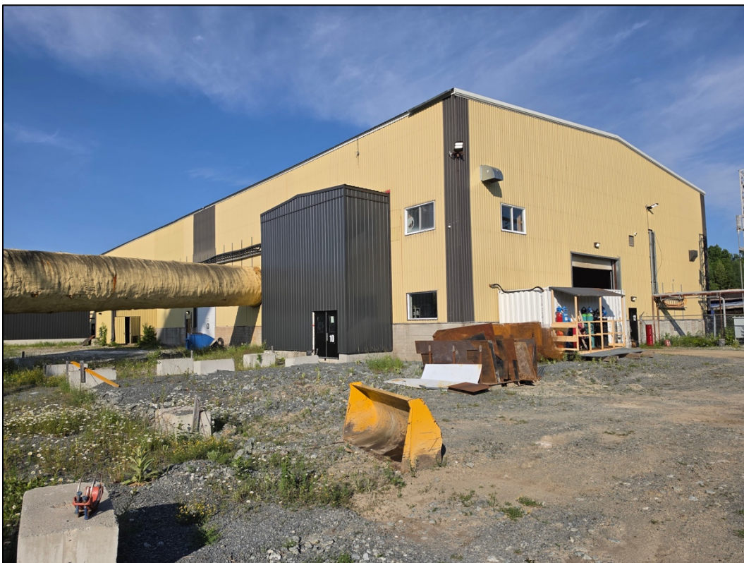
Photo 4: Repainted entrance and staging area for Beacon Mill facility
