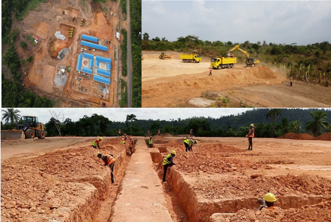
Figure 1: Ongoing construction activities at Segilola. (Source: https://www.thorexpl.com/ ).
