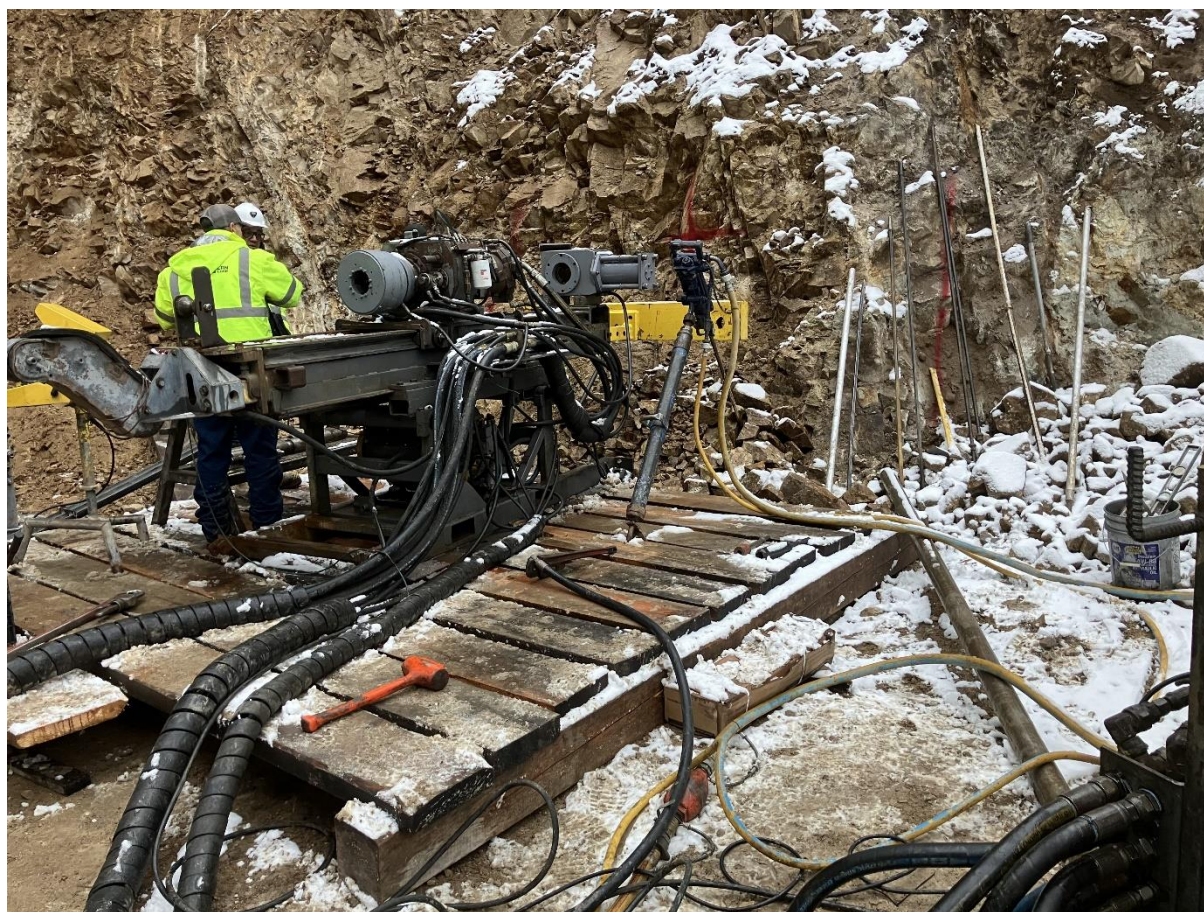
Contract Miner at Face at Washington Mine
