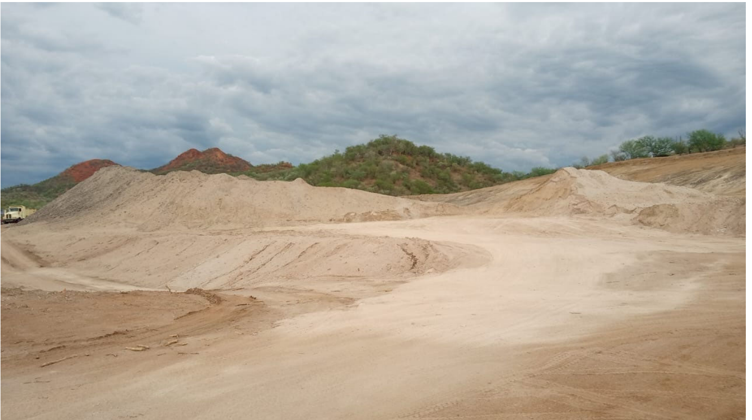
Photo 2. Base for Containment Ponds being packed with clay and ready for liners.
