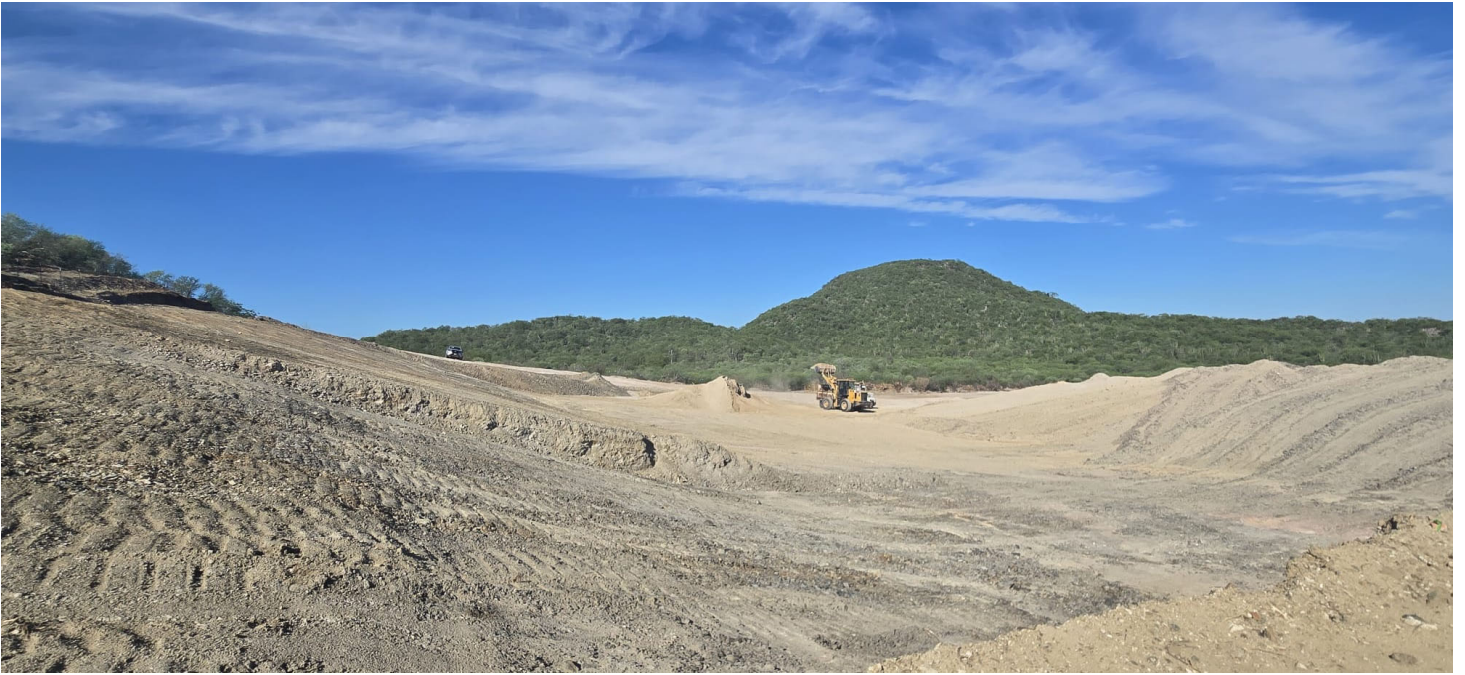
Photo 1. Foundation for Heap Leach Pad excavated and preparing for clay base and liner.
