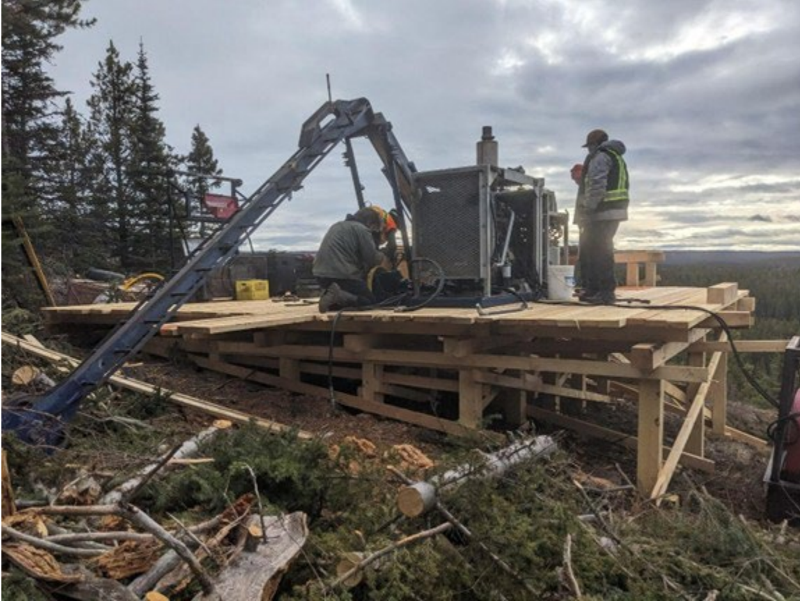
Figure 2-drill installation underway onsite at Star East. Star Copper 2026.
