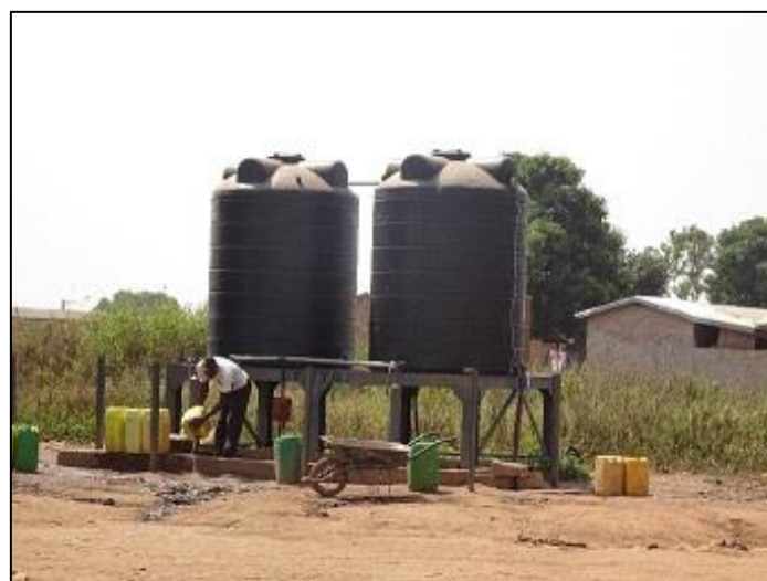
Figure 20-3 Water Tanks at Fadiadougou
