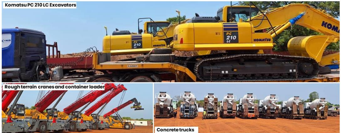
Figure 3: Major earthworks and construction equipment on-site
