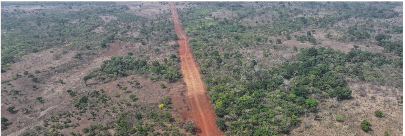
Figure 6: Gbongogo haul road nearing completion
