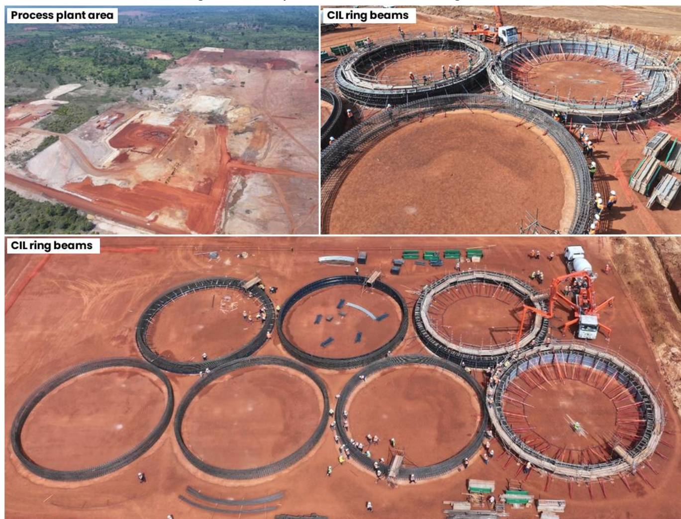
Figure 1: Process plant area overview and CIL ring beams
