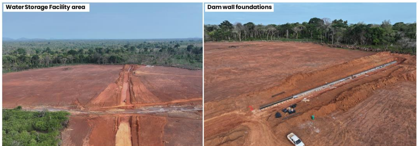
Figure 4: Water Storage Facility preparation
