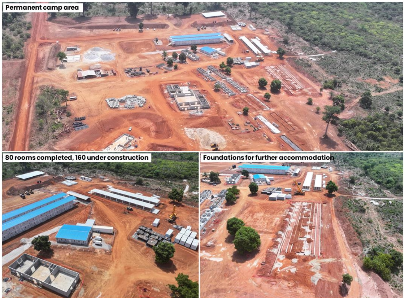
Figure 5: Permanent camp construction progress
