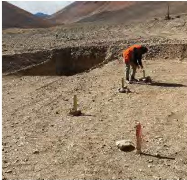
Figure 9.2: Drill Pad Preparation
