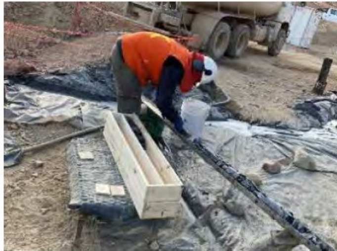
Figure 9.1: Transferring Core to Core Box
