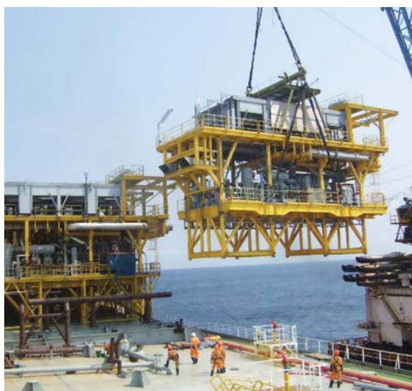
Upgrade of processing facilities on the Espoir field FPSO, offshore Côte d'Ivoire.
