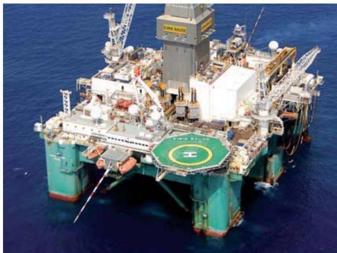
Eirik Raude semisubmersible rig during drilling operations, offshore Côte d'Ivoire.
