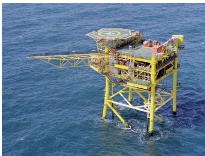
Production facilities on the Ketch field in the UK Southern North Sea.
