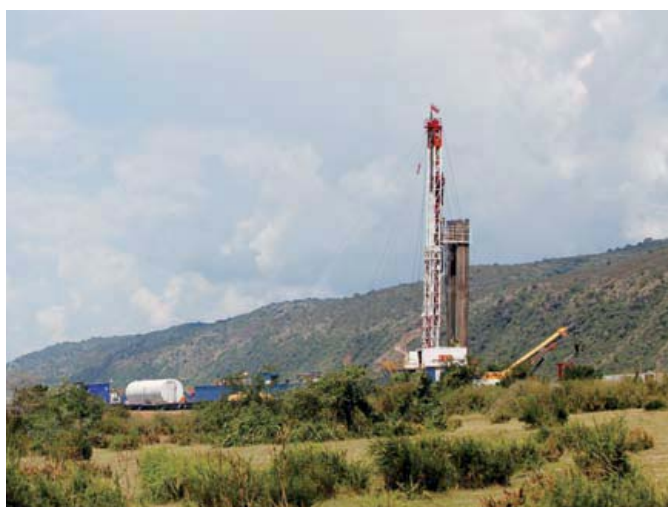
The K900 rig during drilling operations in Block EA-1, Uganda.
