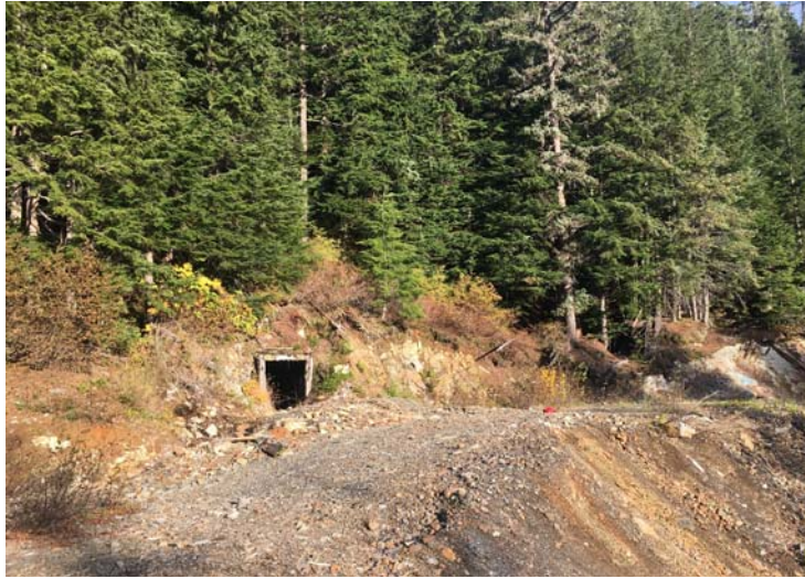
Photo 6.1: Number 4 (Main) Adit
