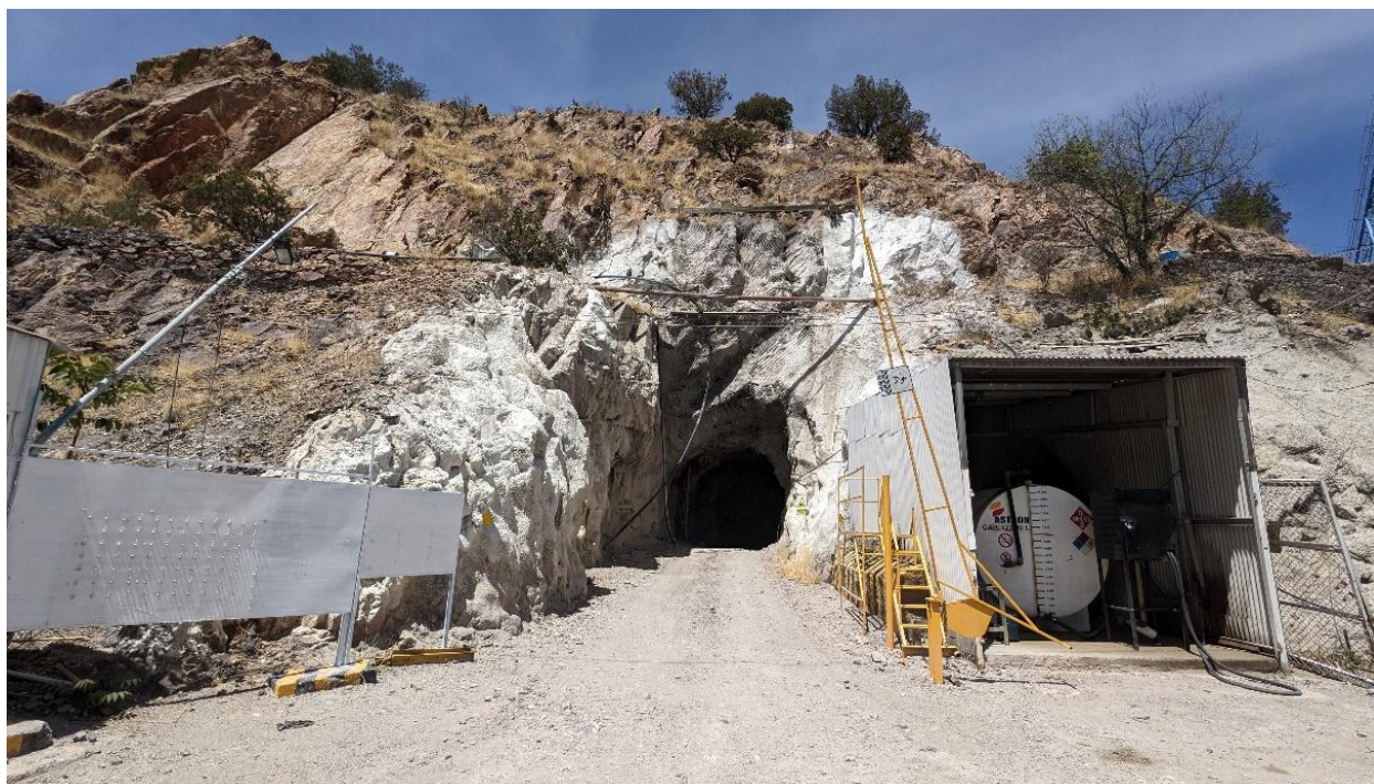
Figure 6-5: Portal to the Promontorio Mine
