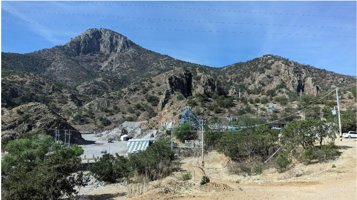
Figure 5-5: Medium Voltage Power Lines Outside the Former Promontorio Mine
